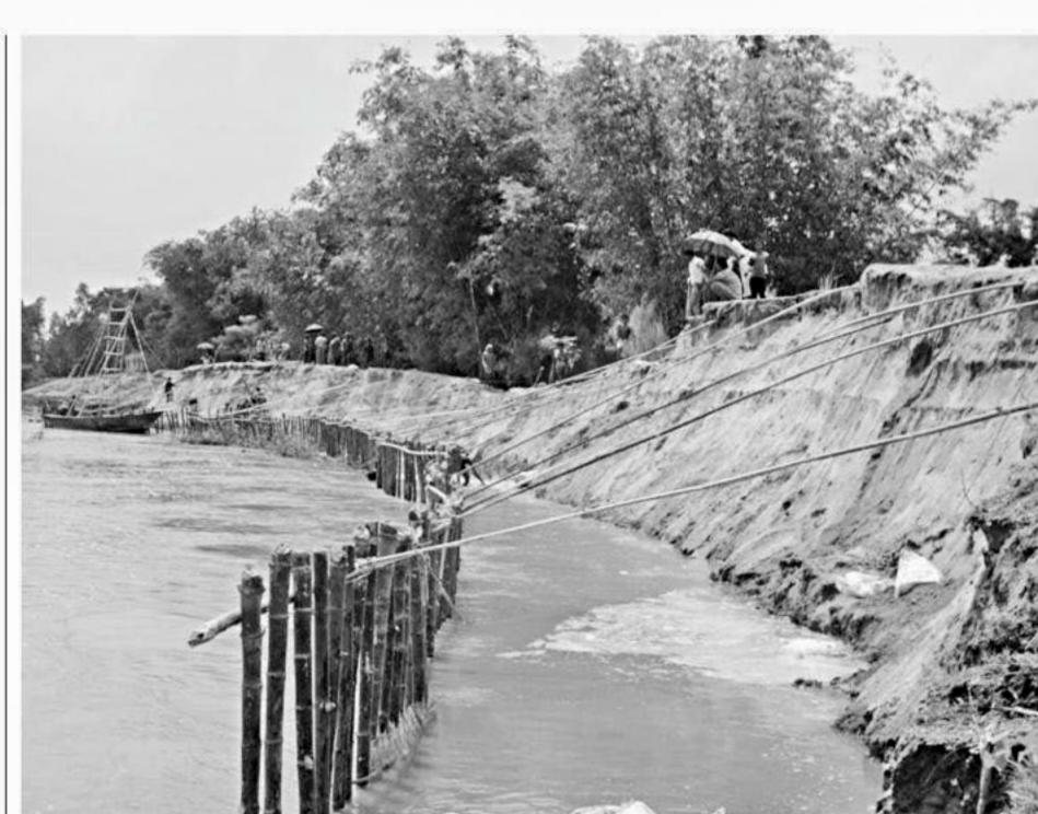
The Teesta has devoured a good portion of the 240-metre stretch of the protection embankment at Uttar Dawabari village in Hatibandha upazila under Lalmonirhat district in the downstream of Teesta Barrage during the last few days, as the bamboo spars and sandbags put by the villagers failed to stop the erosion.
