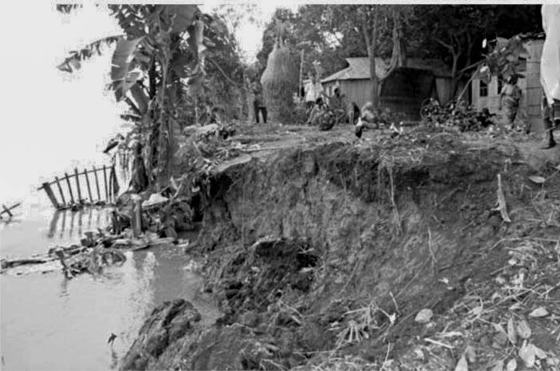
Erosion by the Brahmaputra River has taken a serious turn, threatening around 800-metre area of an embankment at Saroktari village in Raniganj union of Chilmari upazila under Kurigram district.
