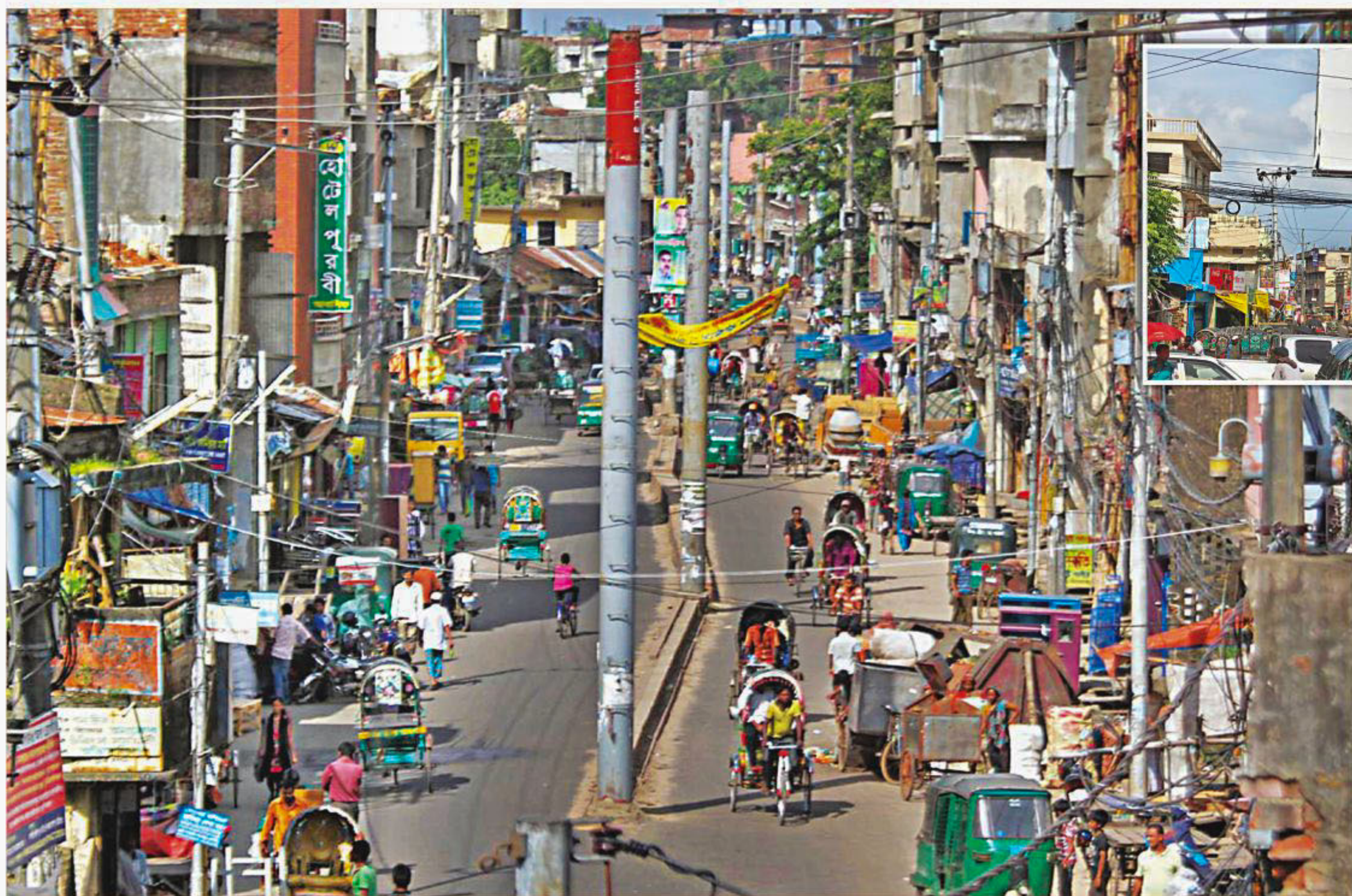
Illegal pillars, meant to house billboards, erected by breaking down a newly constructed road divider on a road being upgraded to four lanes in Pathantuli area of Chittagong city. Inset, some of the pillars already have billboards with contact numbers for those who wish to put up ads there. The photos were taken recently.
