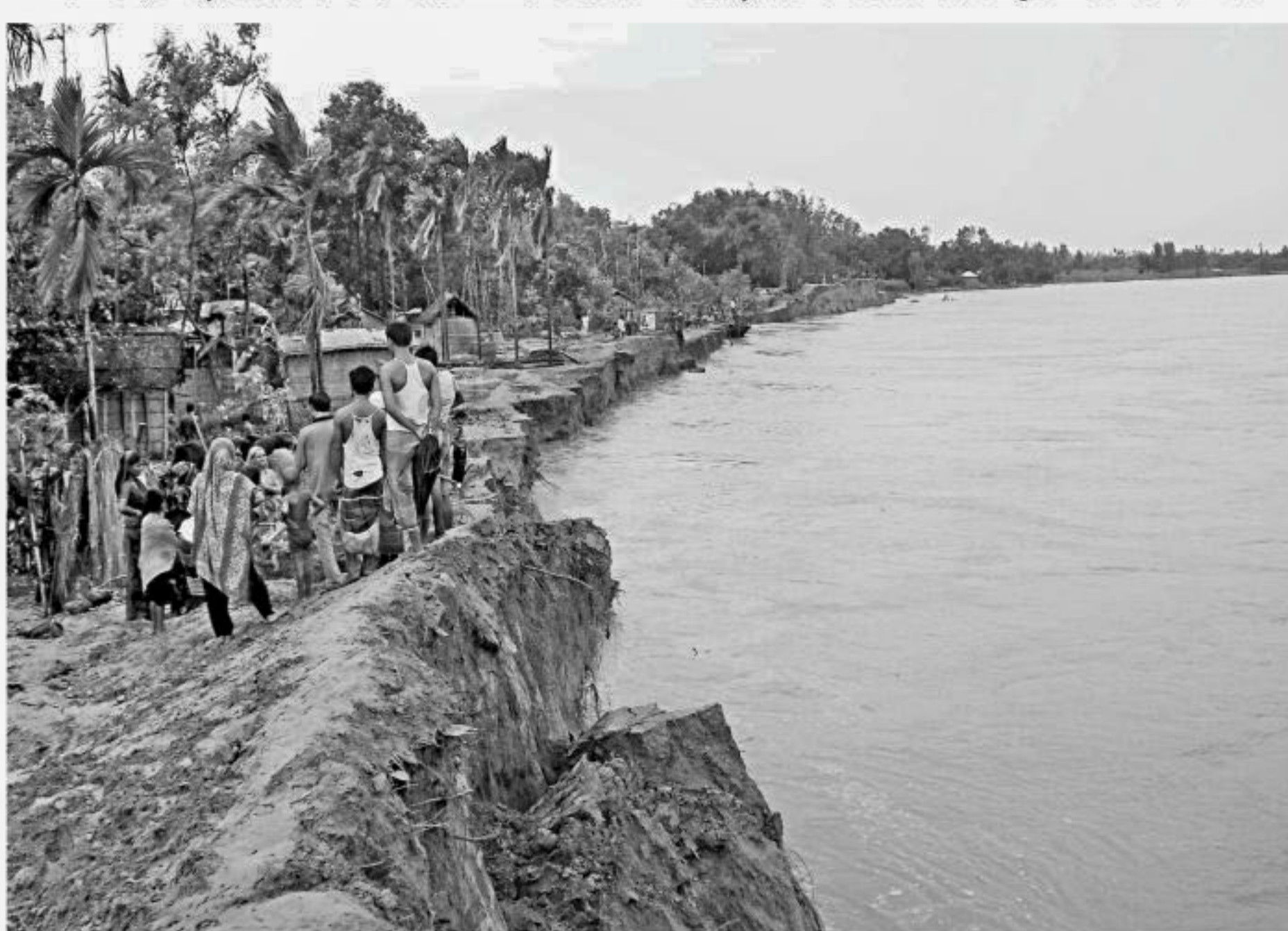
Erosion by Brahmaputra washed away about one kilometre of the flood protection dyke and rendered around 300 families homeless in a week at several villages under Jatrapur union of Kurigram.
