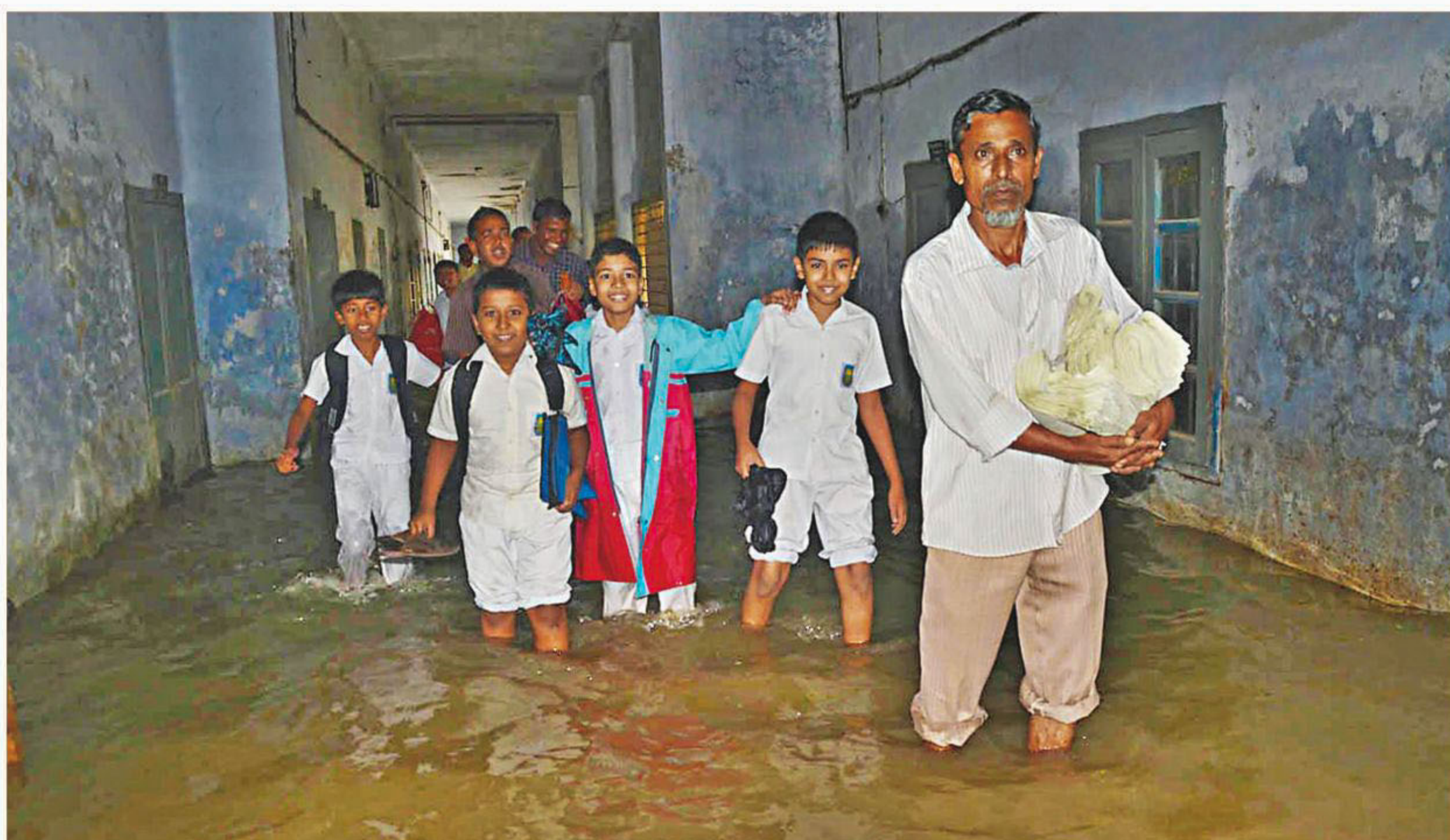
Flooded Bakalia Government High School's building in Chittagong city with its students and staff wading through knee-deep water yesterday following heavy downpour that battered the city from around midnight on Saturday till yesterday morning.
