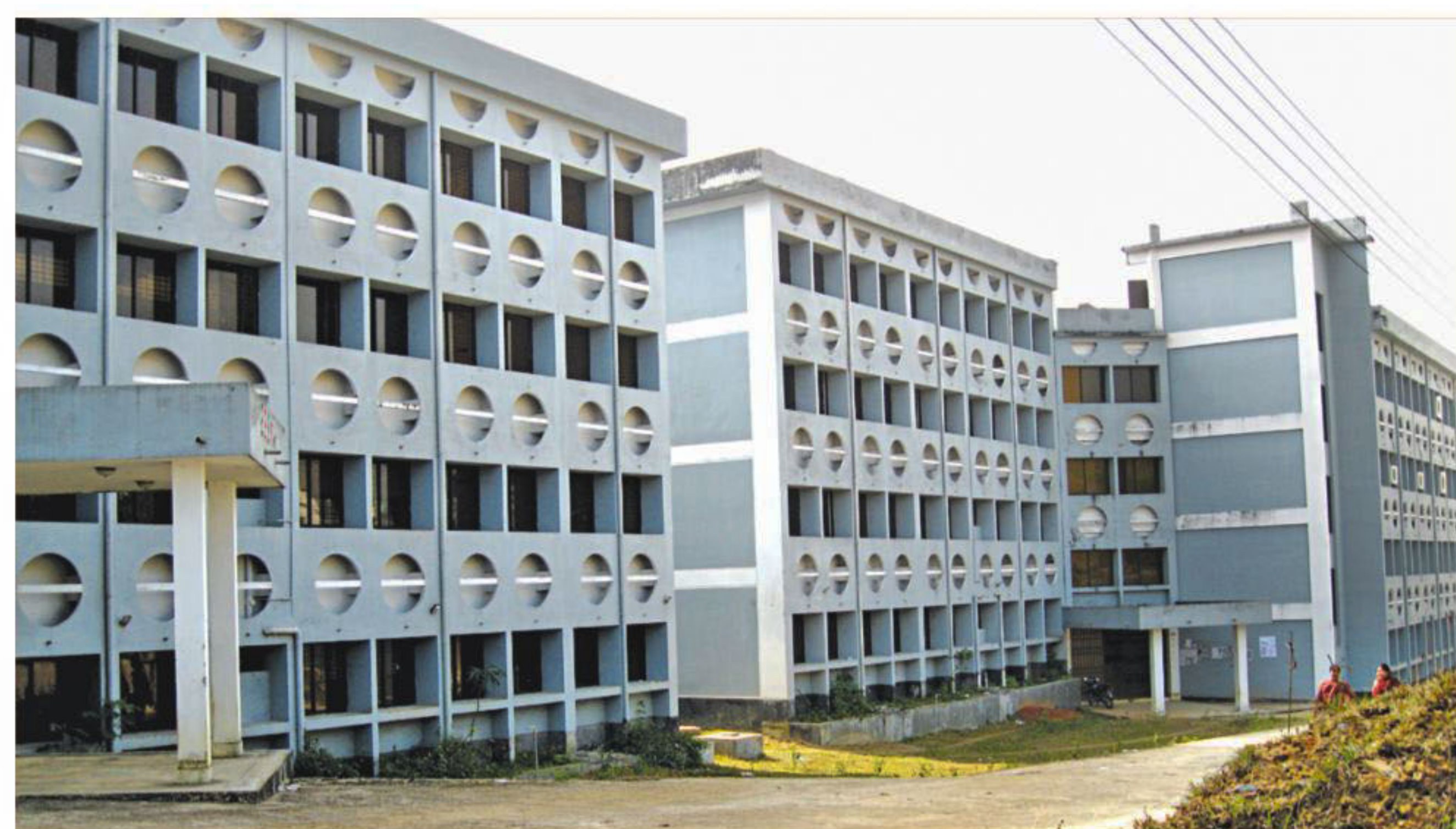
Two huge buildings of Sylhet Engineering College, located just outside Sylhet city, lie in disuse since its inception in 2006 because of absence of teaching faculty. Only 12 visiting teachers are running one of the three departments while the two other departments do not have any students enrolled. The photo was taken recently.
