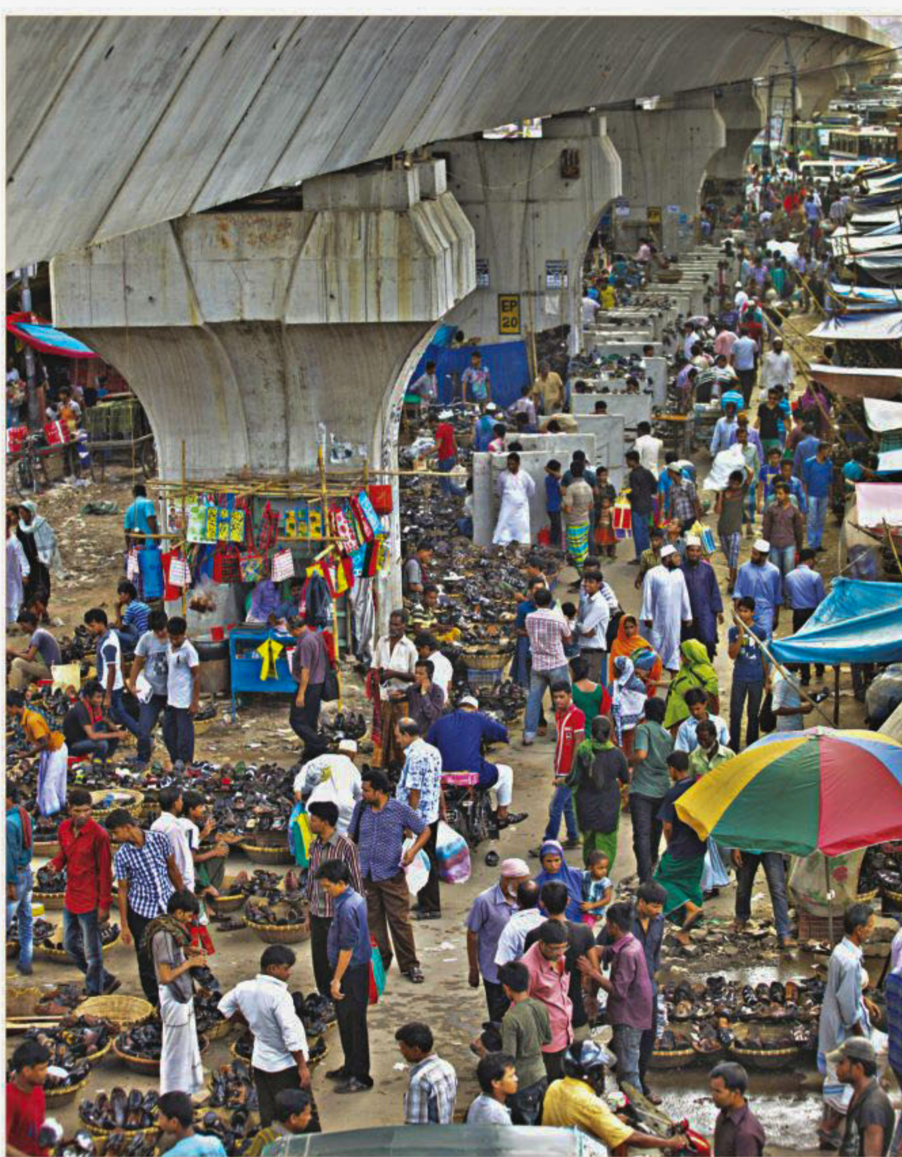
Street vendors have set up shops under the under-construction Gulistan-Jatrabari flyover at the capital's Gulistan, ignoring the risk of accidents anytime. The numbers of both vendors and shoppers have increased lately ahead of Eid-ul-Fitr. The photo was taken yesterday.
