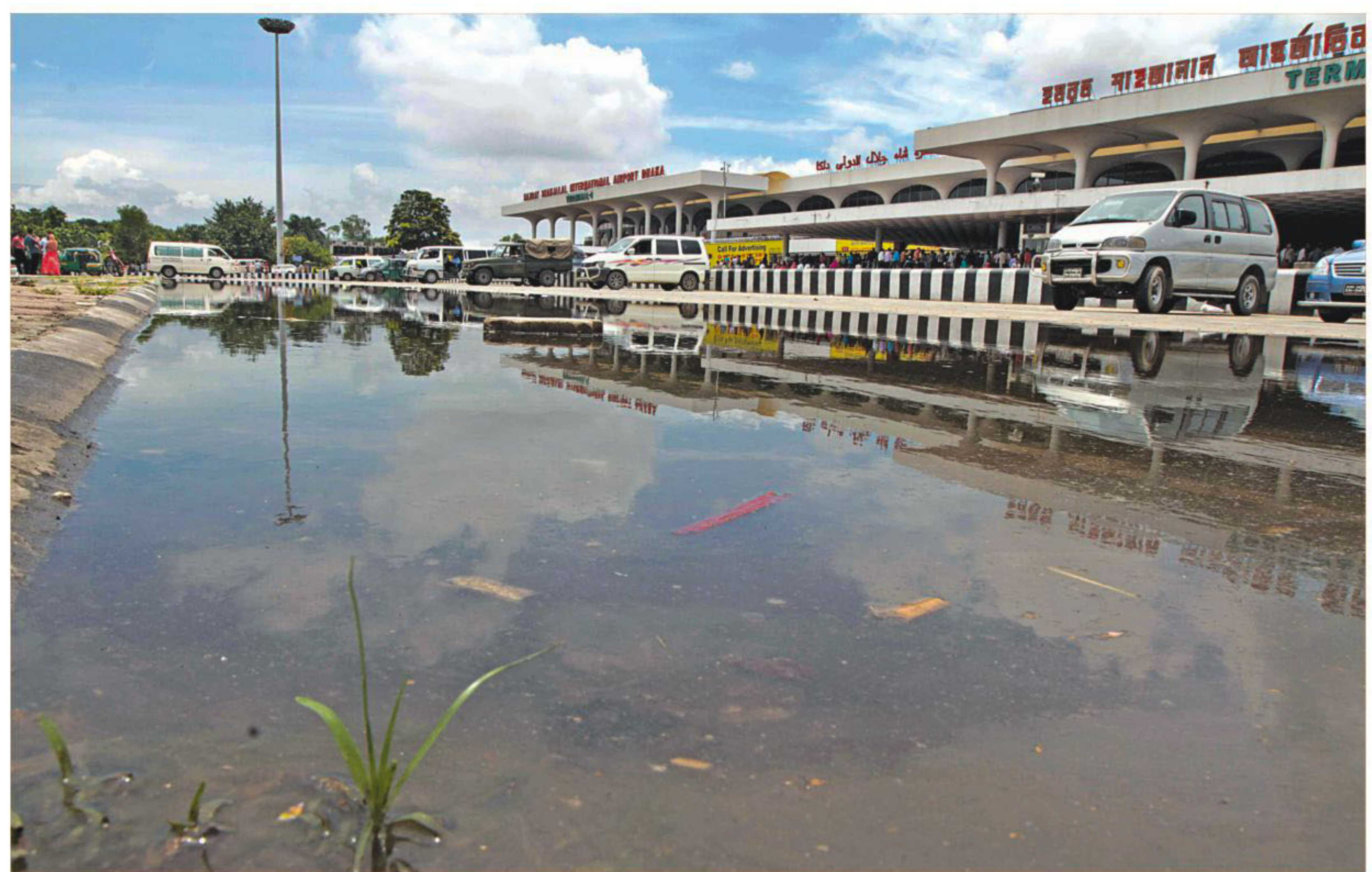
A waterlogged parking lot in front of Hazrat Shahjalal International Airport in the capital. The car park gets inundated as it does not have a proper drainage system. The photo was taken recently.
