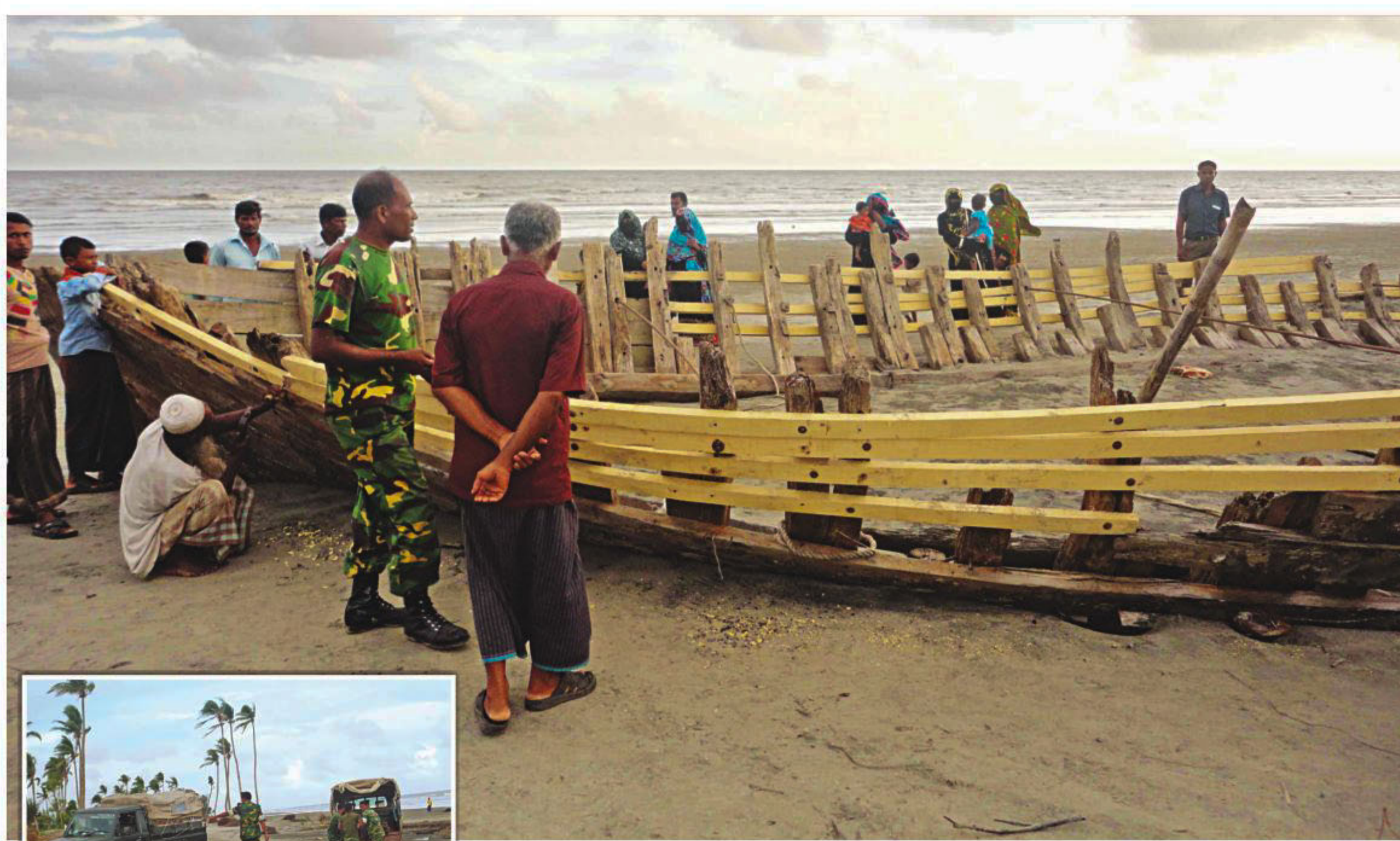
The ancient sail ship which surfaced on Kuakata beach in June last year undergoing some primary repair works under the supervision of an army team yesterday. Inset, army men unloading wood planks which will be laid like rail tracks to wheel out the boat to its preservation site three kilometres away.
