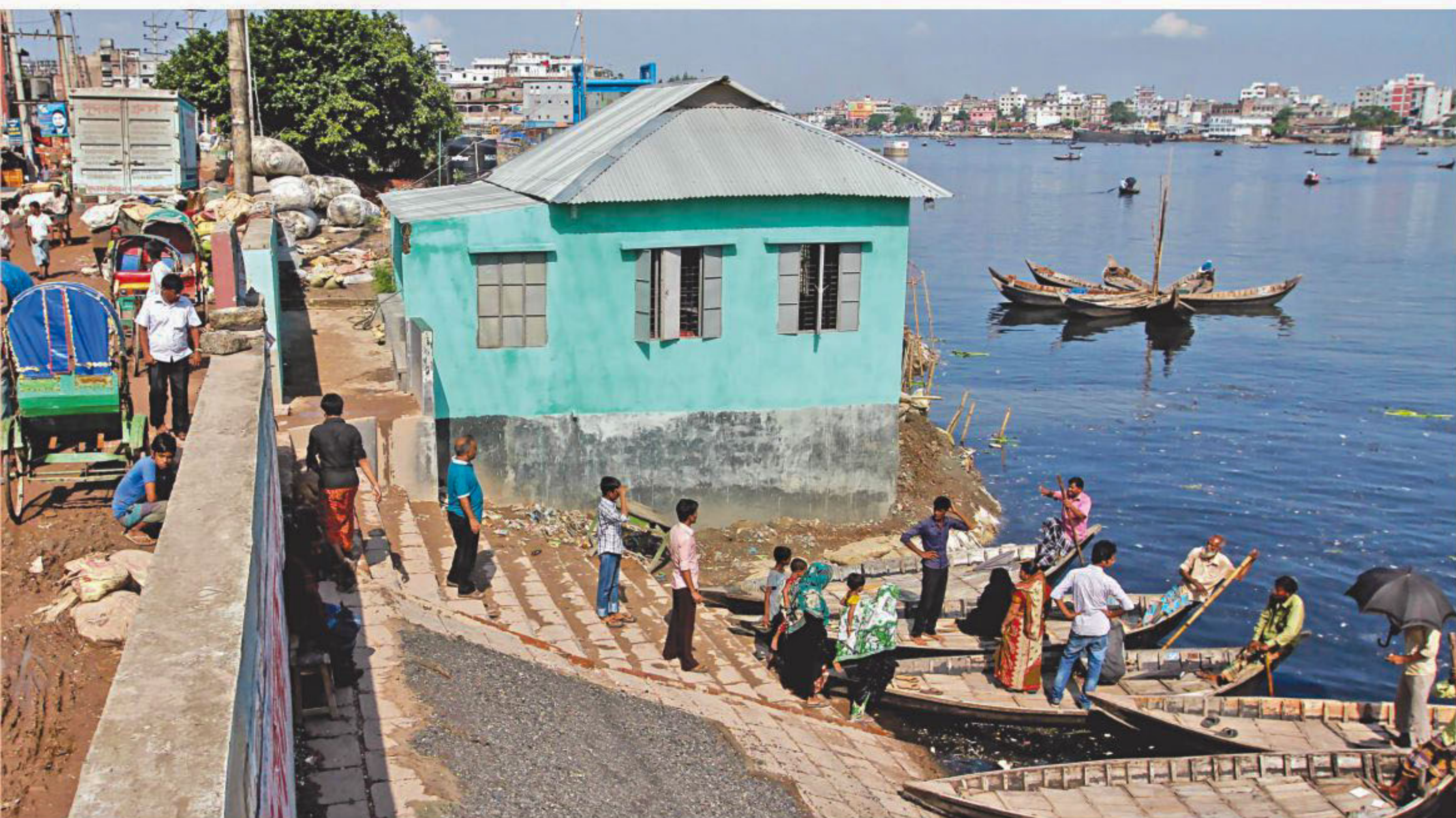
The South Islambagh Panchayet Committee has erected its office through encroachment of a part of the river Buriganga. Although it claims to be a non-political organisation, local leaders of the ruling alliance are reported to be involved with it. The photo was taken yesterday at Islam Alir Ghat, Lalbagh.
