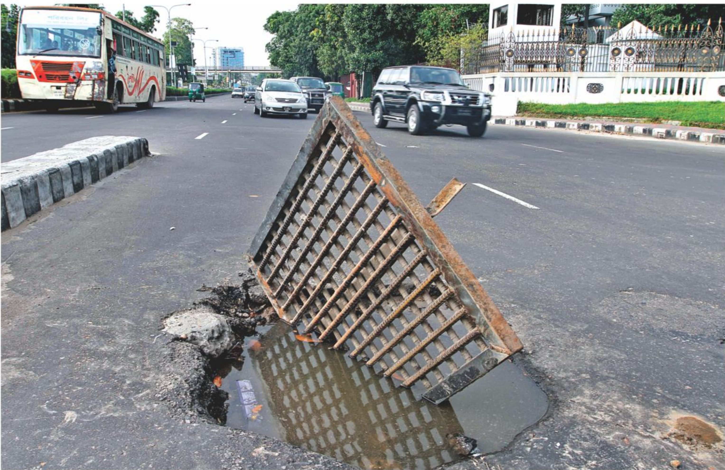
The cover of a storm-water drainage line breaks and sticks out. Motorists could easily not see the danger and an accident could happen, as there is no warning sign. Interestingly, the photo was taken yards away from the Prime Minister's Office on one of the better-maintained thoroughfares of the capital.
