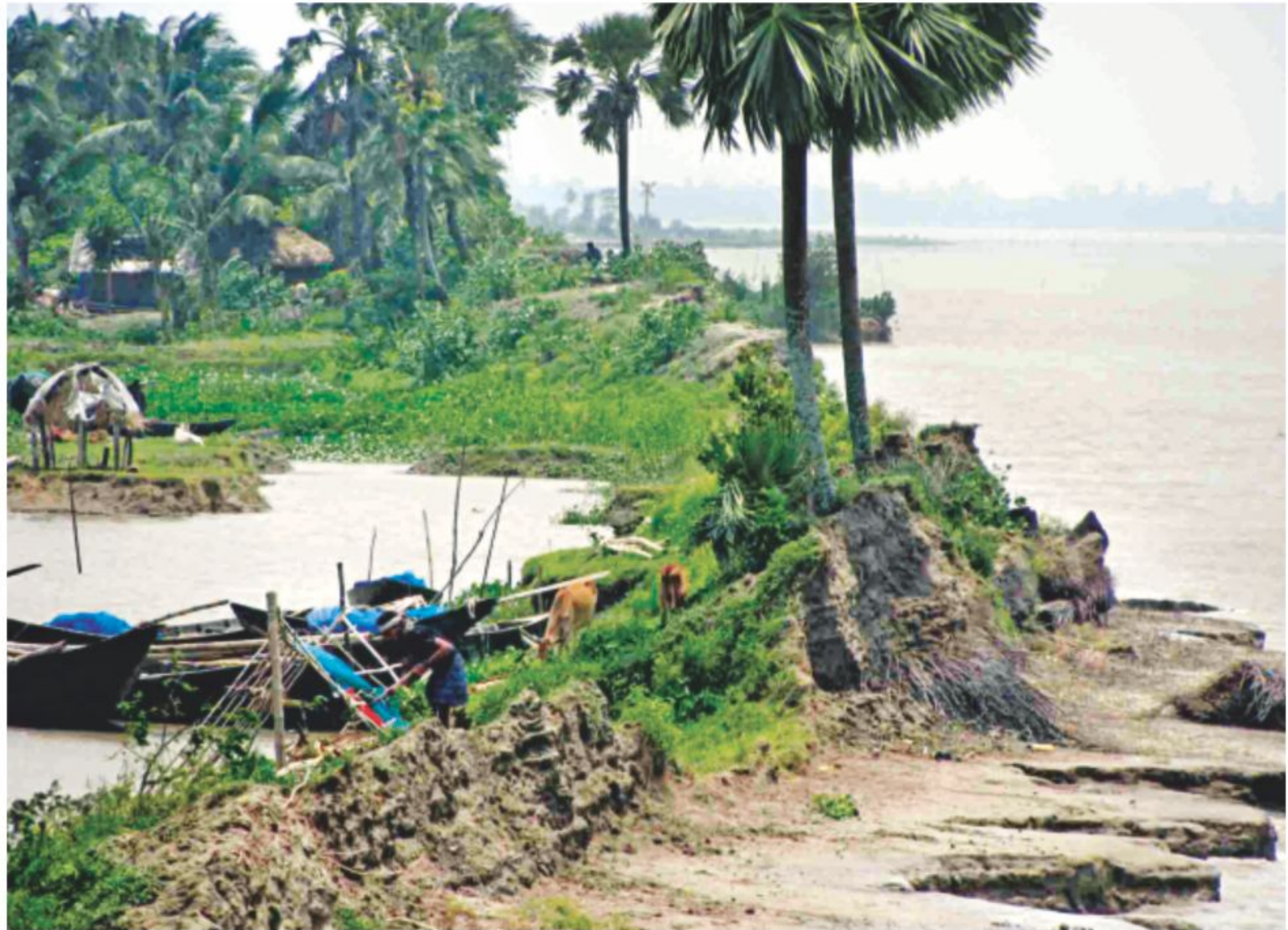
Left without any repair after serious damage by super cyclone Sidr on November 15 in 2007, this embankment on the Kacha River in Mathbaria upazila under Pirojpur district cannot save the nearby villages from flooding even during moderate rise in the water level of the river.
