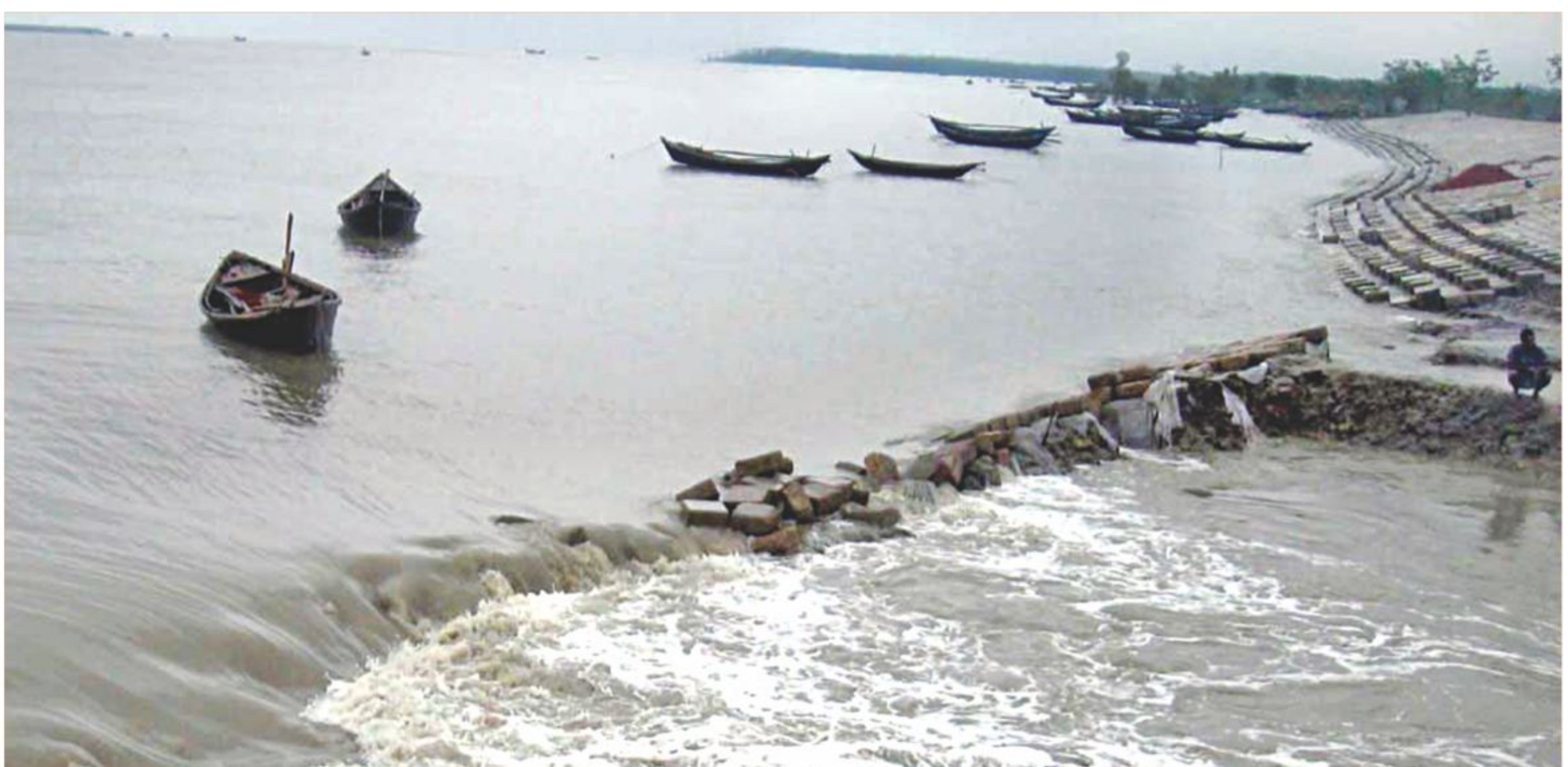
Water gushing into villages through a breach in the flood protection embankment along the River Andhar Manik at Sudhirpur in Patuakhali's Kalapara upazila. Cyclone Mahasen on May 16 damaged the embankment.
