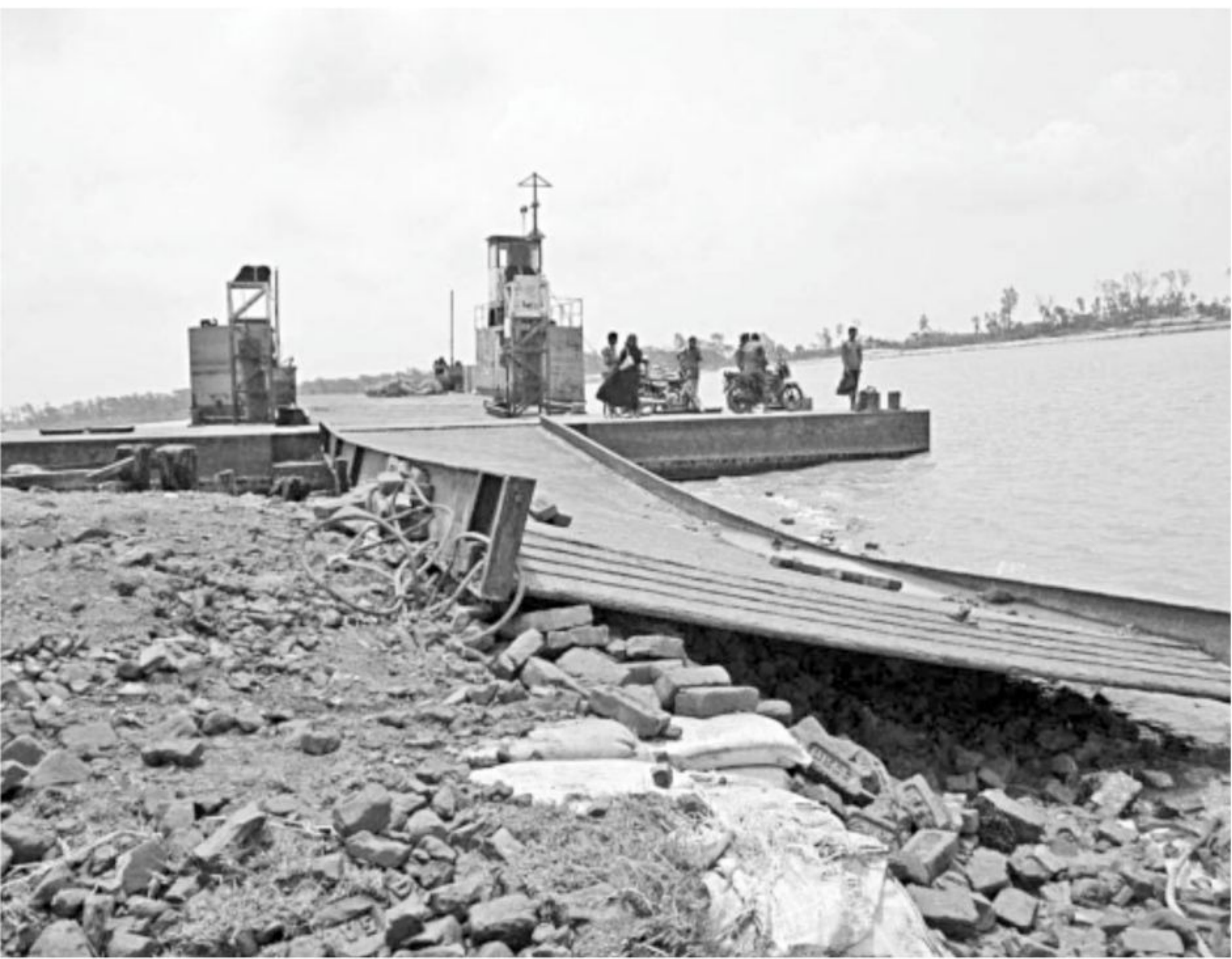
Transport of vehicles through Baliatali ferry terminal on the alternative road of Patuakhali-Kuakata highway has remained suspended for the last five days as the pontoon and the gangway were thrown onto the bank during the onslaught of cyclone Mahasen on Thursday.
