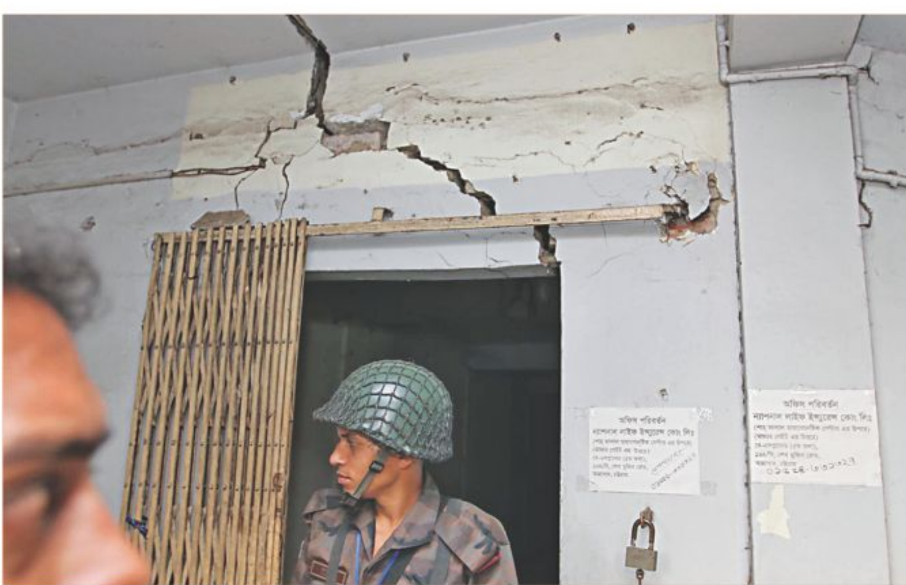
Cracks are seen on the concrete walls of JACKS Shopping Complex in the port city of Chittagong. A mobile court finally sealed the building.
