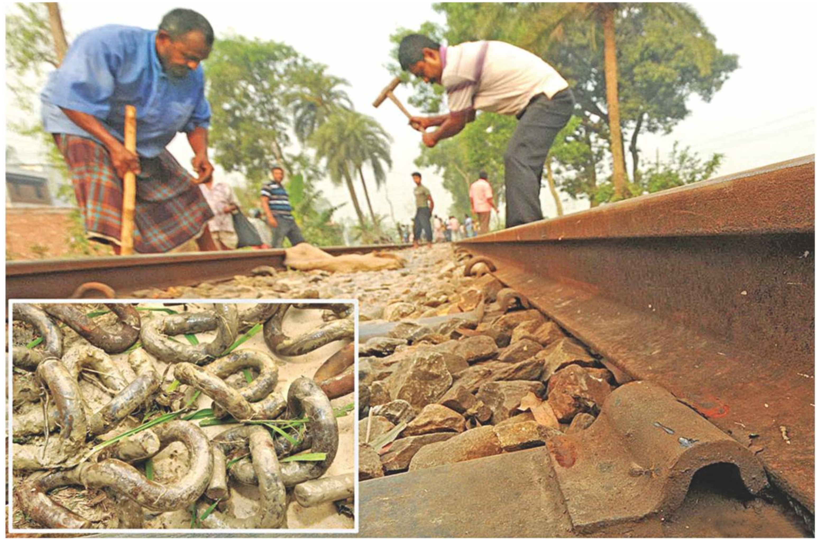
Criminals early yesterday removed 945 clips holding the rail lines to their sleepers in Bogra. Inset, some of the removed clips.
