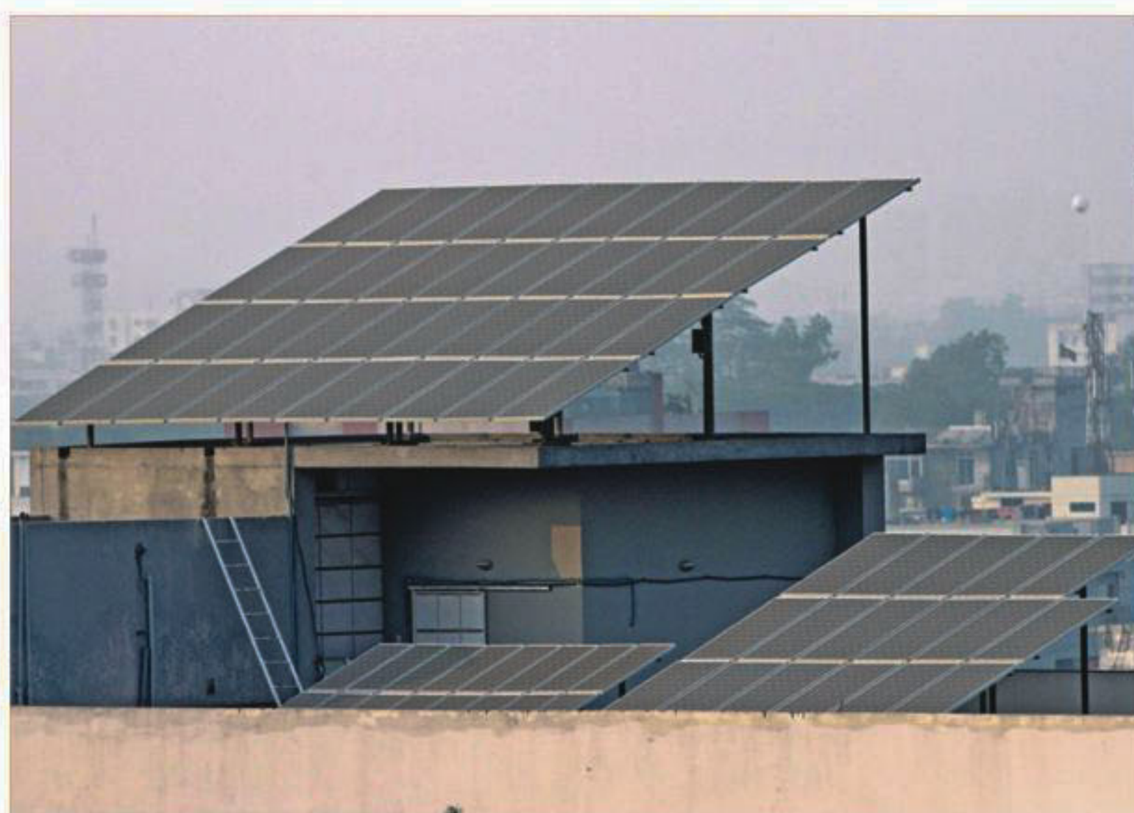
STAR A solar home system sits on a rooftop. More than 50,000 solar home systems are installed a month, according to the World Bank.
