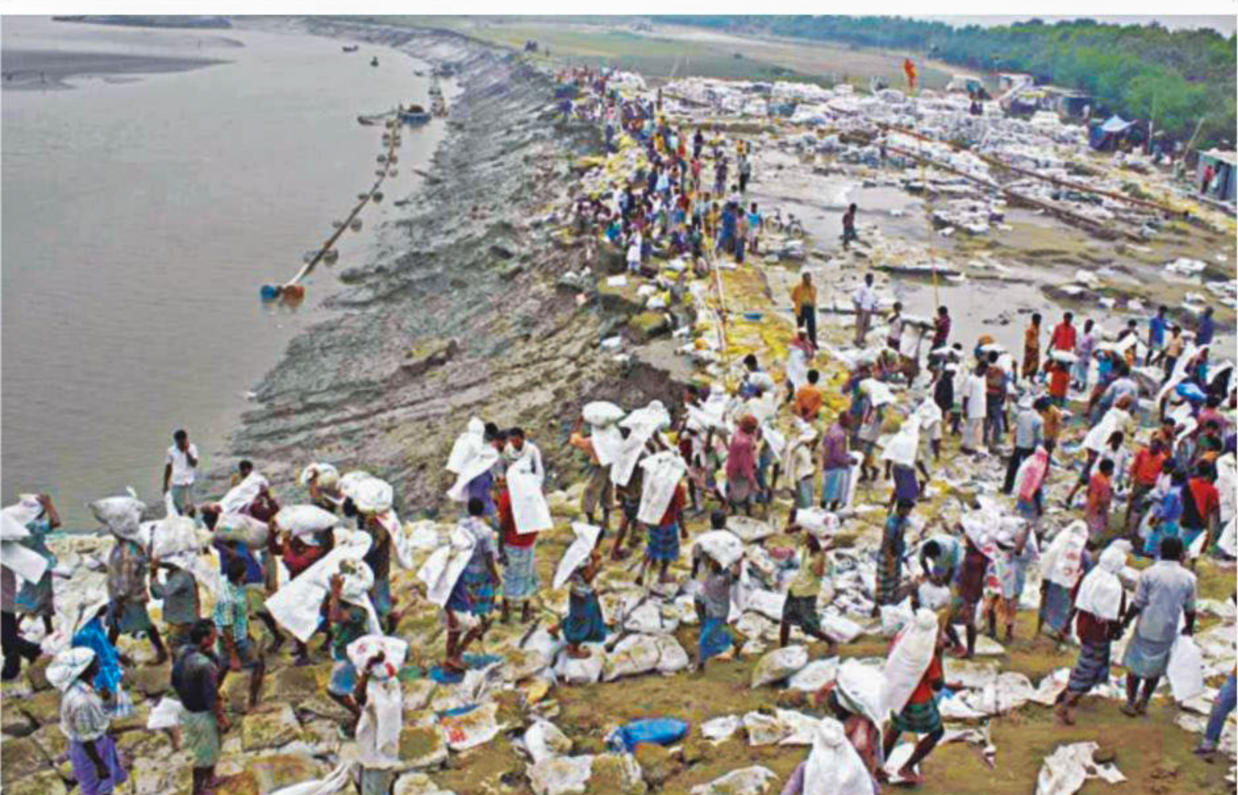
PHOTO: STAR The water Development Board (WDB) authorities completed the 'closure dam' on Feni River in Char Chandina area yesterday afternoon. Built under a Tk 10 crore project, the dam, however washed away in just 3 hours at 6:00 pm due to strong tidal surge. The photo was taken moments before the completion of the dyke.
