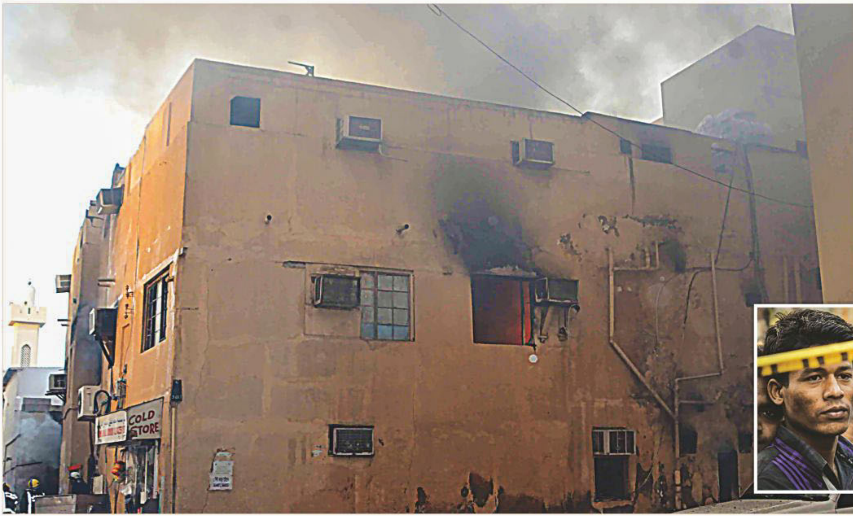
Smoke billows from a burning building that houses Asian workers, mostly Bangladeshis, in the Bahraini capital Manama on Friday. Inset, migrant workers stand behind a police cordon as firemen and rescue workers inspect the building.
