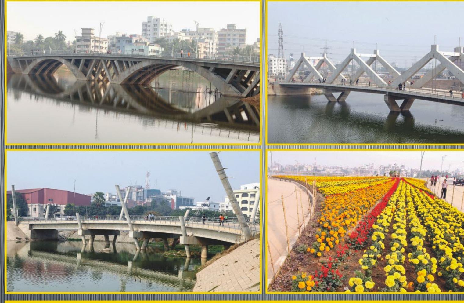
BSRM is proud to be associated with this Landmark Project of the Capital City having supplied the reinforcing steel Xtreme500W conforming to BDS ISO 6935-2:2009 Grade 500WC to the project.
