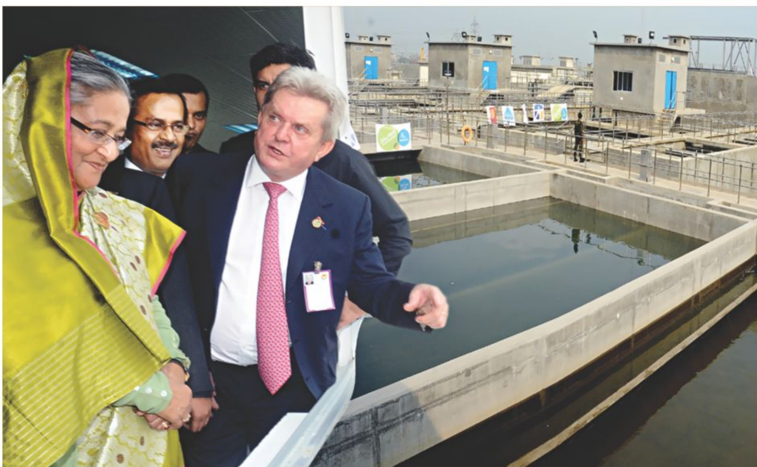
Prime Minister Sheikh Hasina goes around the Sayedabad Water Treatment Plant phase-II after commissioning the new phase of the plant in the capital yesterday. With the launching of the new phase, the plant's capacity will be doubled from 22.5 crore litre a day and there will be no water crisis in the city, claims Dhaka Wasa. Story on page 2.
