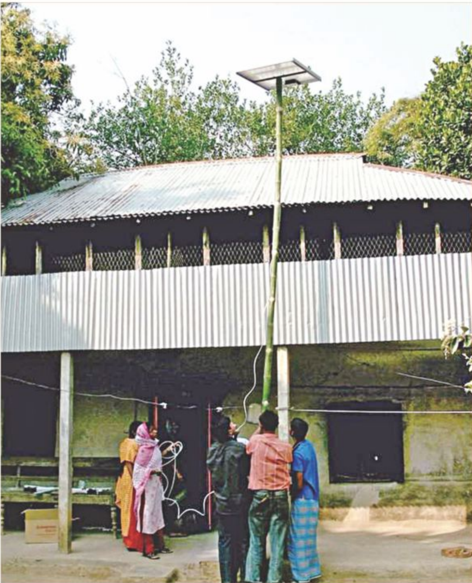
People install a solar panel, which is a great source of power in off-grid areas.
