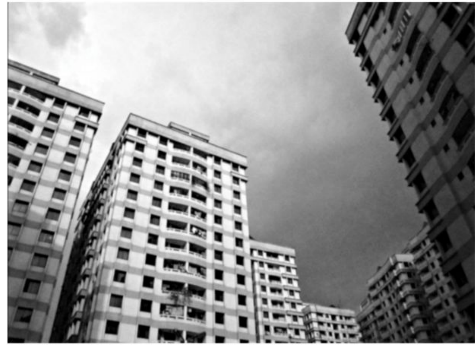
Not following the directives related to the surroundings of a site including keeping open space. PHOTO: STAR
