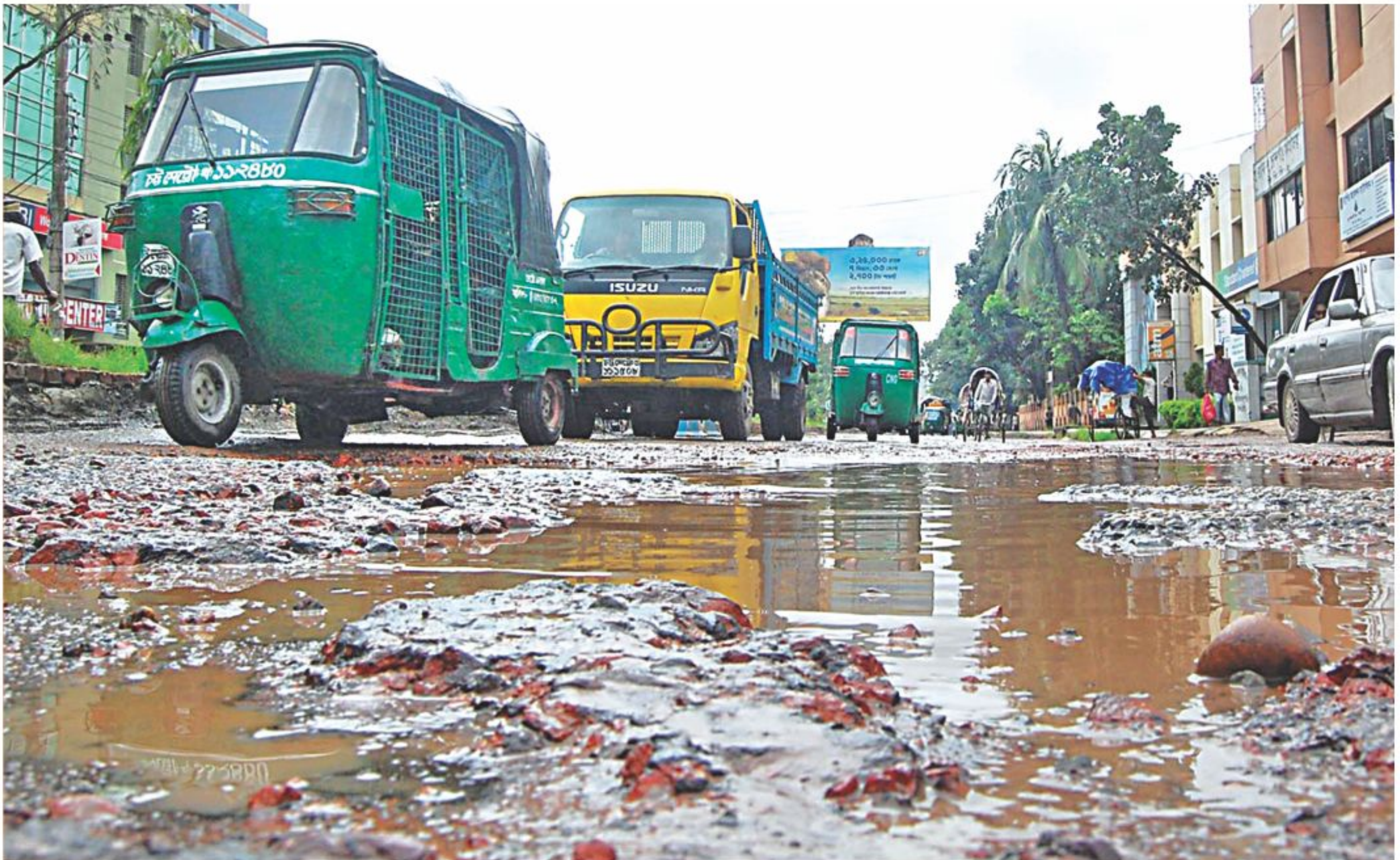
Arakan Road, one of the major thoroughfares in Chittagong, has been in bad shape for years owing to an absence of repair or maintenance. Commuters find it an ordeal travelling on this potholed road every time it rains. The photo was taken yesterday.
