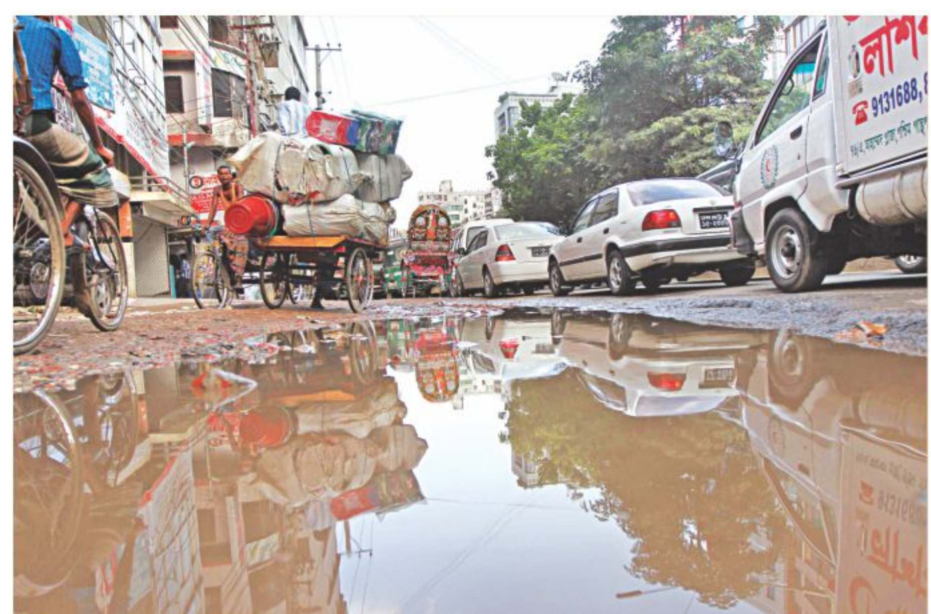
Muddy puddles and potholes make vehicular movement difficult over this portion of road near the intersection connecting Panthapath, Russel Square, Karwan Bazar and Farmgate in the capital as patches of the road dug up for utility works were not covered up afterwards. The photo was taken yesterday.
