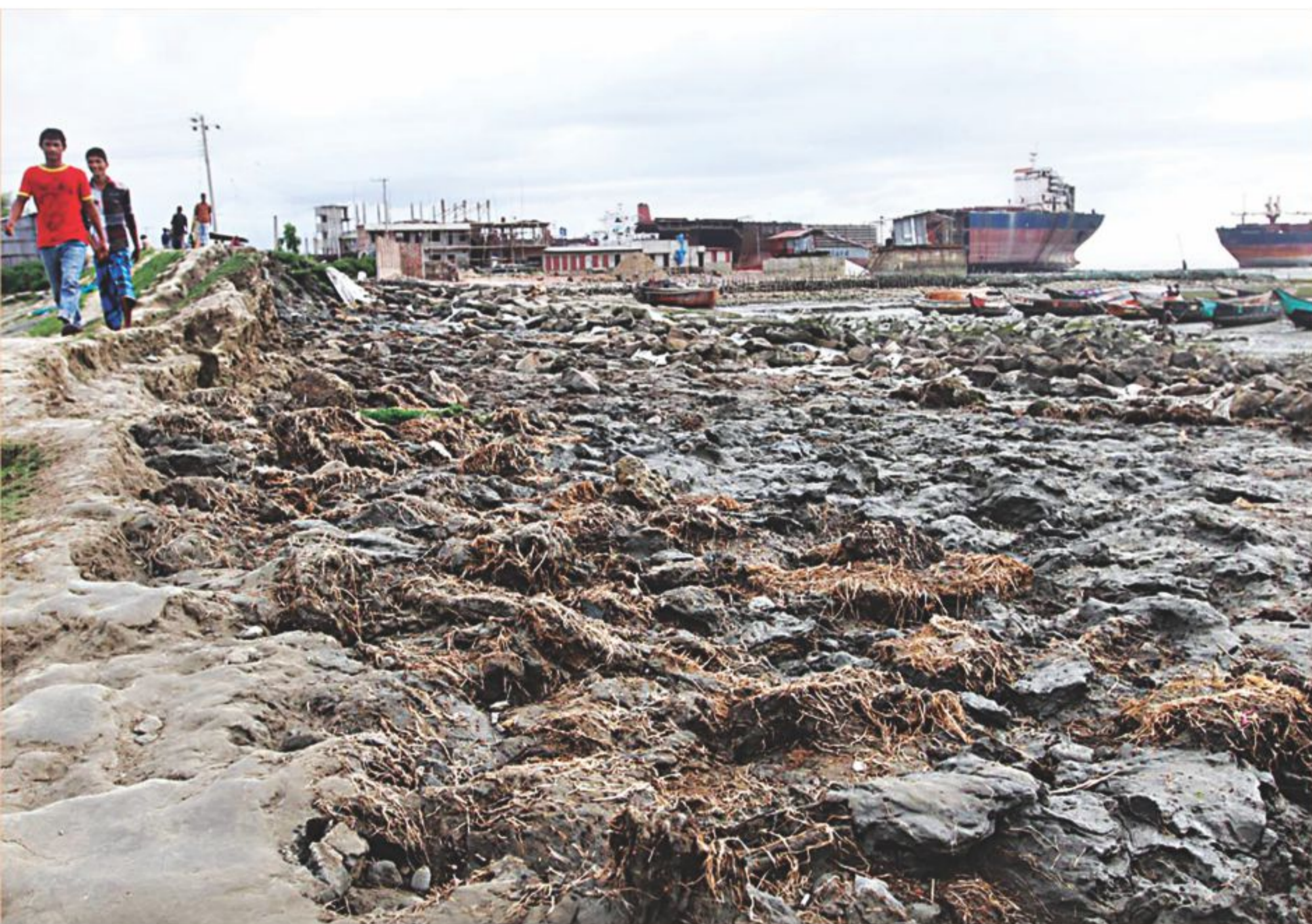
The embankment of Sonaichhari union at Sitakunda upazila of Chittagong being eroded away by the Bay of Bengal. Locals and forest officials blame felling of trees for establishing ship breaking yards as the reason behind the erosion. The photo was taken recently.
