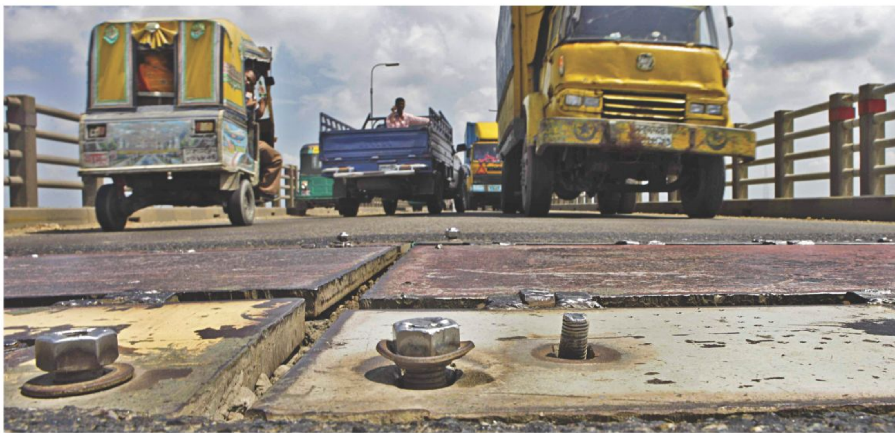
Nuts and bolts of the temporary expansion joints at Meghna-Gumti bridge are seen protruding in a photo taken on Sunday. The authority has to monitor the bridge round the clock and readjust them every time it is required.
