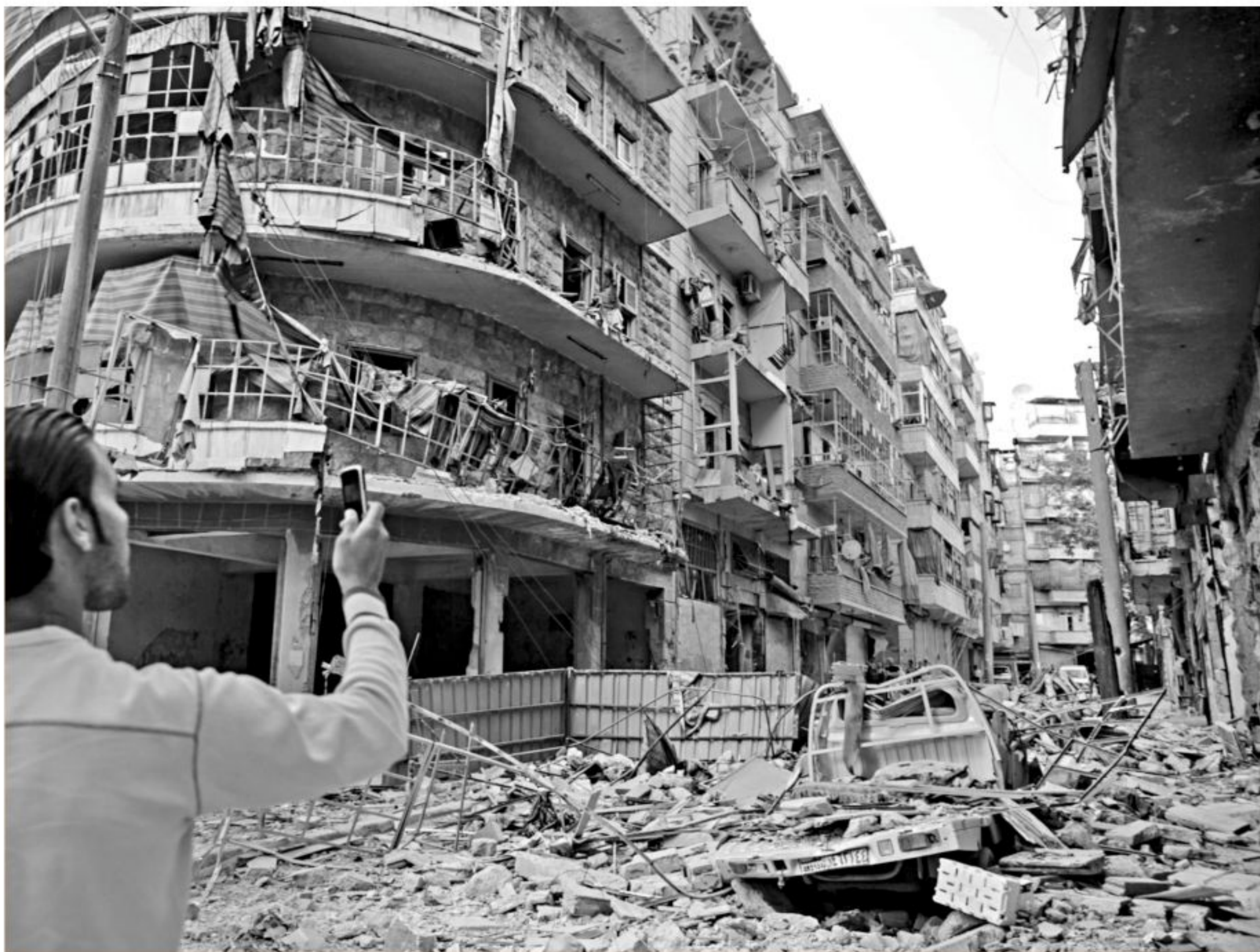
A Syrian man takes pictures with his mobile phone of damage caused by aerial bombardment from government forces in the neighbourhood of Tariq al-Bab in the northern Syrian city of Aleppo on Tuesday.
