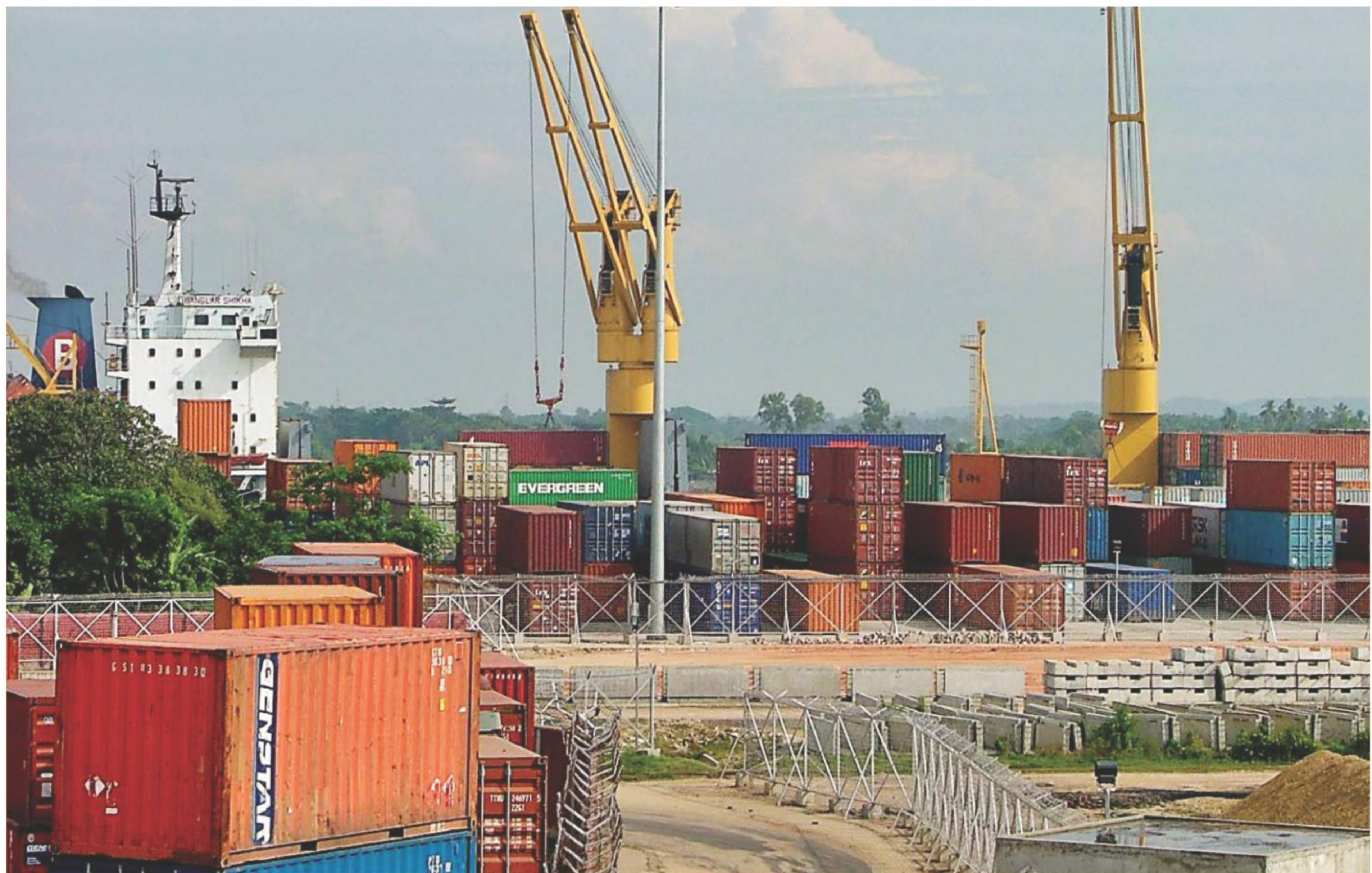
The newly built New Mooring Container Terminal of the Chittagong Port. The terminal has remained idle since it was built in 2009, affecting the overall functioning of the prime seaport.
