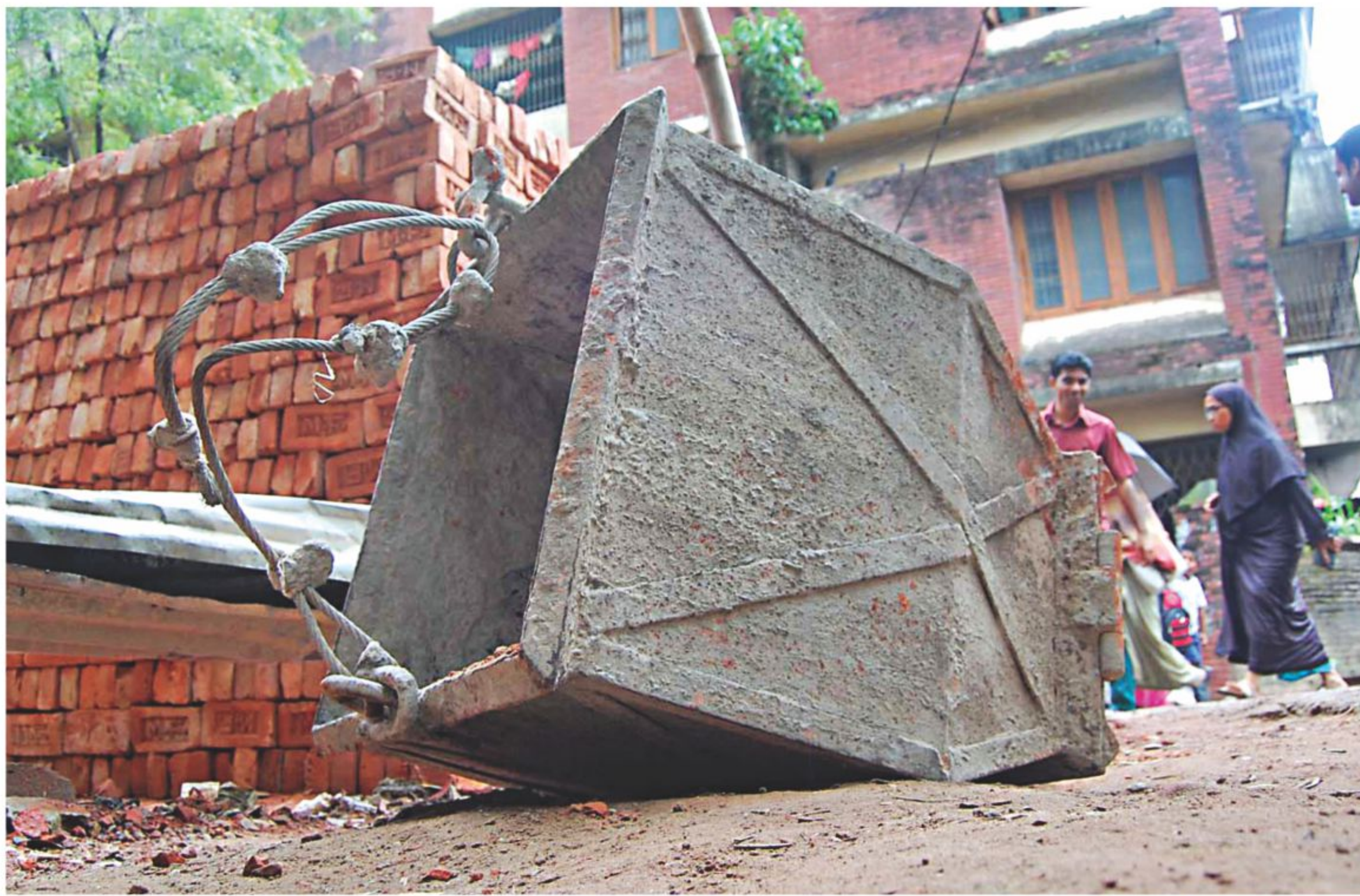
A passerby narrowly escaped when this heavy construction equipment fell yesterday morning from a 10-storey under-construction building of Baytech Real Estate at Dewanji Pukurpar of Chittagong city.
