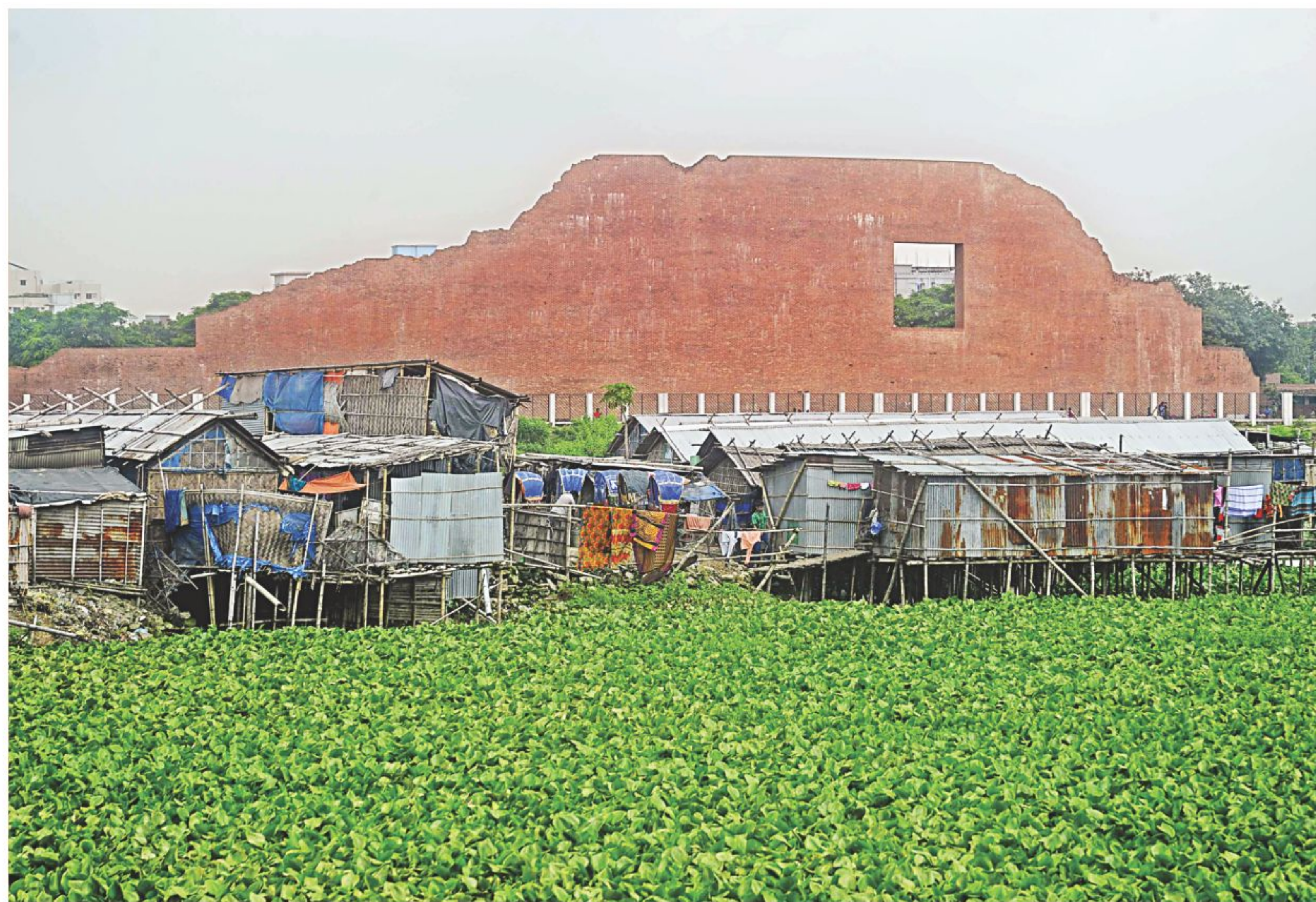
The ambience surrounding the Martyred Intellectuals' Memorial in the capital's Rayerbazar seems to be degrading with time. Squatters have set up makeshift structures all around, an adjacent canal has been narrowed down by encroachers and criminal activities spiral with almost non-existent security measures in the area. The photo was taken yesterday.
