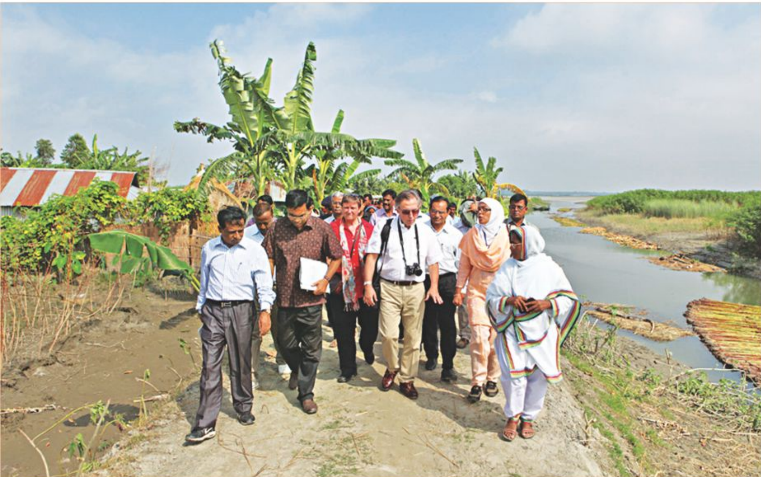
Charge d'Affaires of Brazil in Bangladesh Fausto Godoy and UN's World Food Programme Representative in Bangladesh Christa Rader, along with Local Government Engineering Department engineers and local representatives, are walking a newly constructed road doubling as an embankment at Char Barovita, a shoal in the Brahmaputra river, in Chilmari, Kurigram. The photo was taken on Tuesday.
