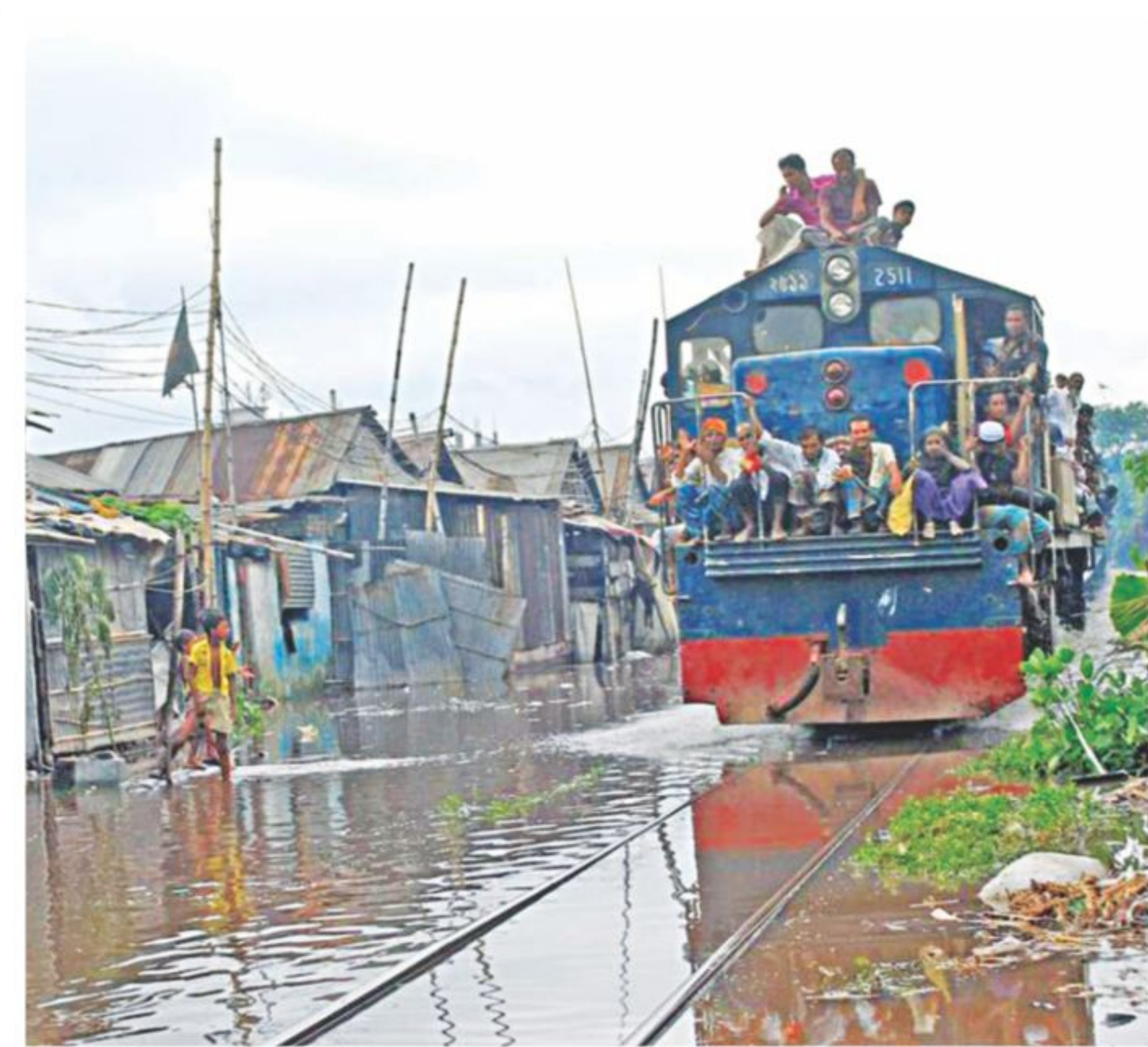
A train on Narayanganj-Dhaka route moves on the tracks submerged in water near Gandaria Railway Station after yesterday's downpours. The area gets waterlogged every time there is a downpour.
