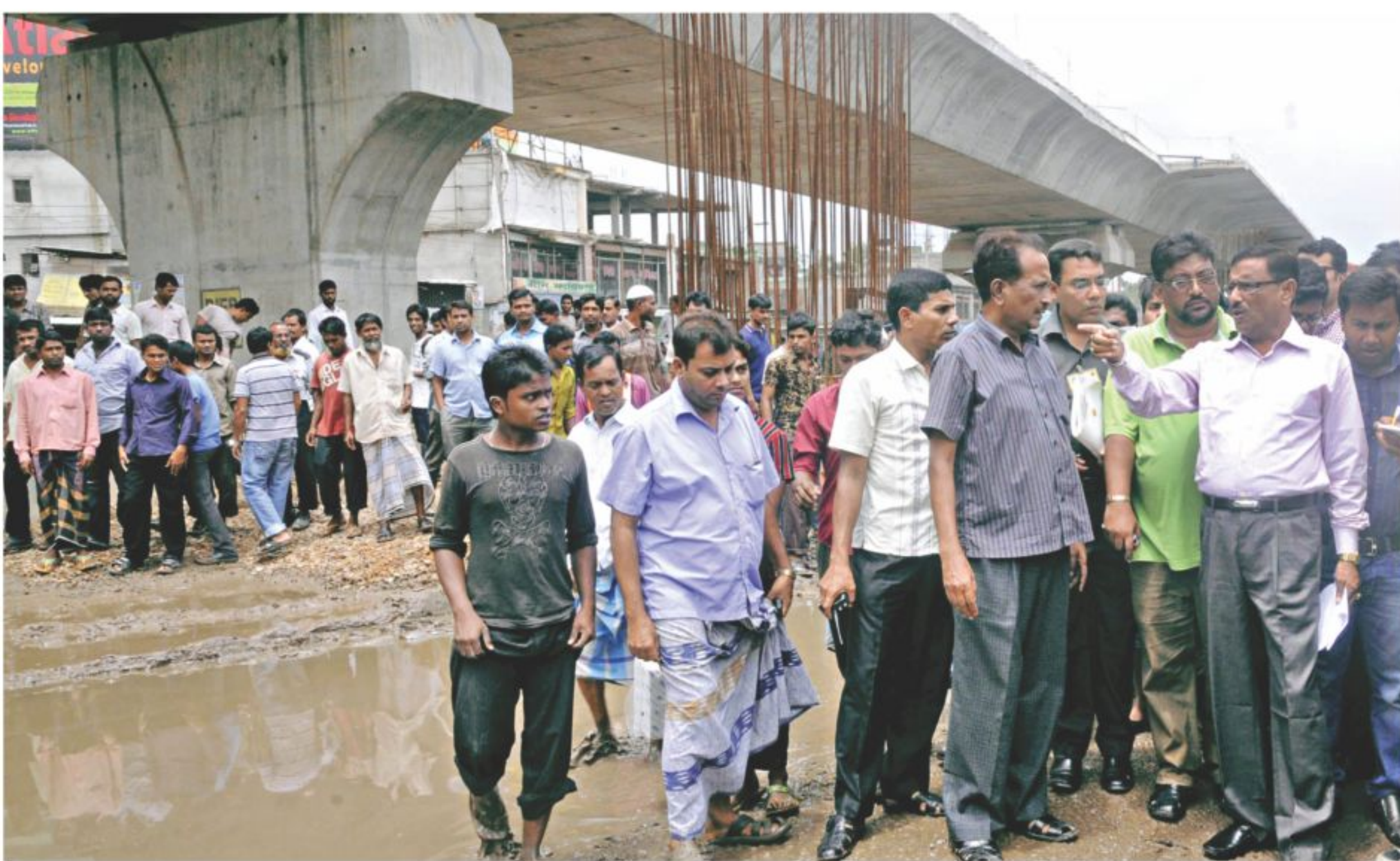
Communications Minister Obaidul Quader visiting the under-construction Mayor Hanif Flyover, and a road, which is in battered condition, in Jatrabari yesterday.
