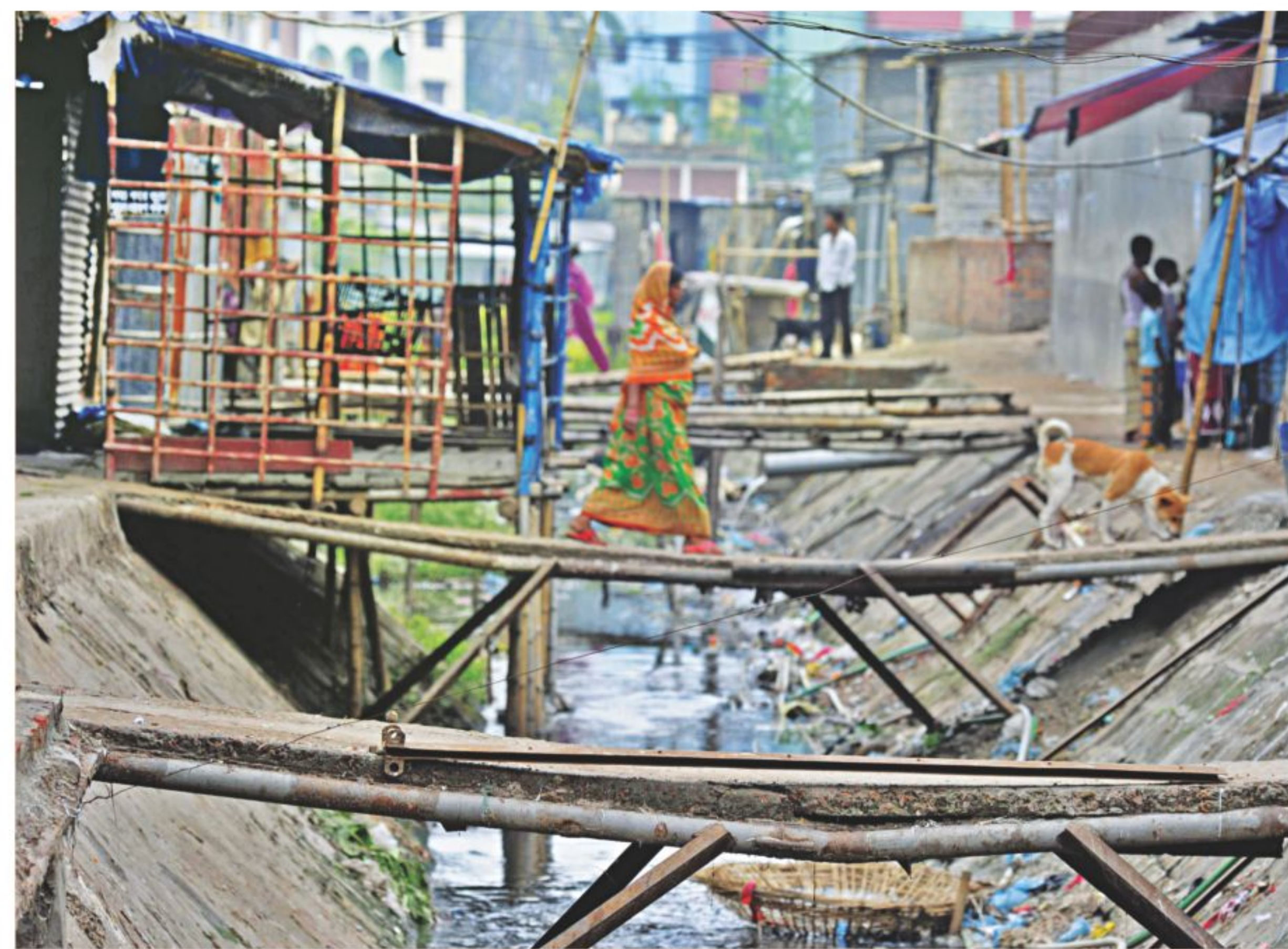
Although Dhaka Wasa knocked down illegal structures over the Mohammadpur canal near old Kazi Office in Shyamoli a few months back, new structures were built over the canal soon after. The photo was taken recently.
