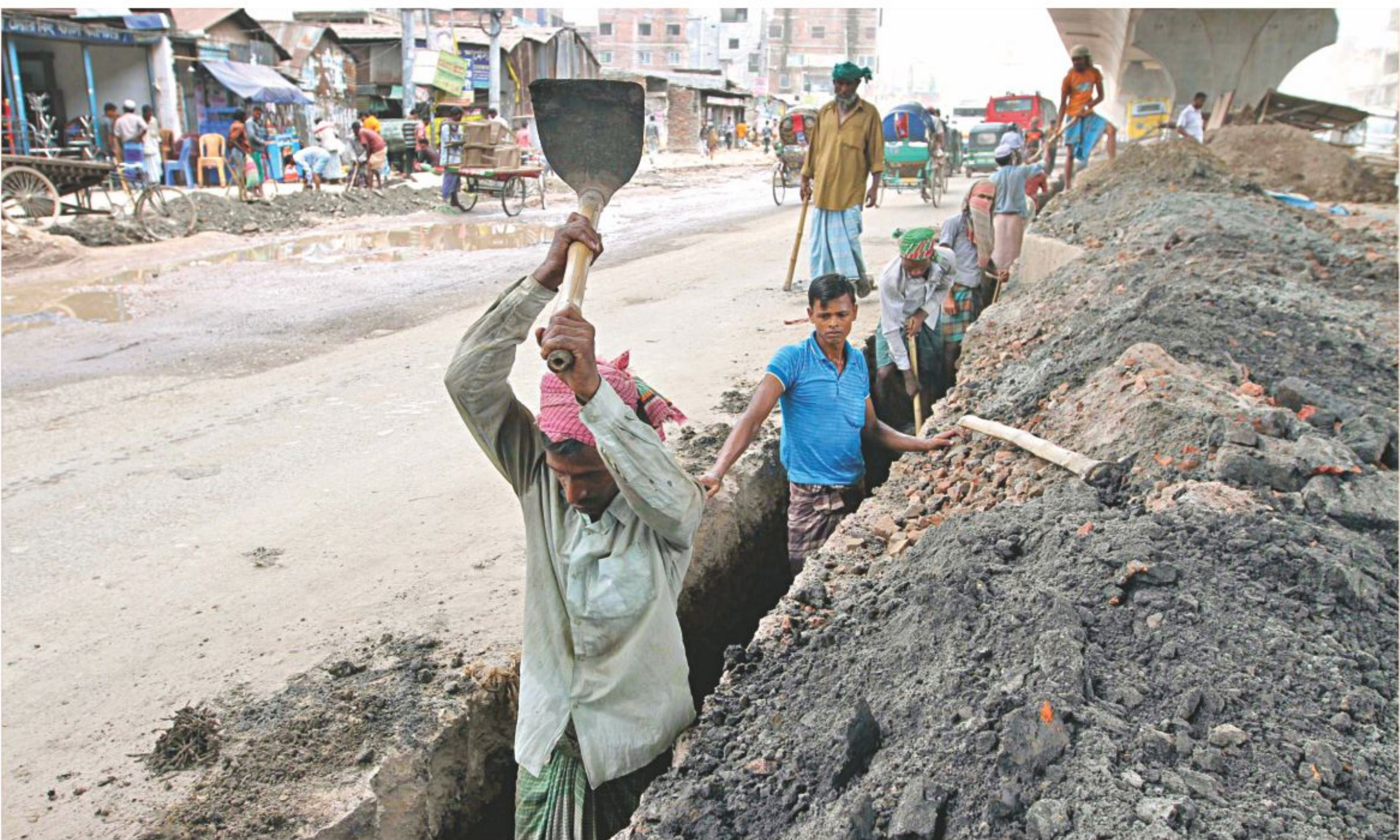
Workers dig a trench for laying utility lines near the under-construction Jatrabari-Gulistan flyover in the capital yesterday.
