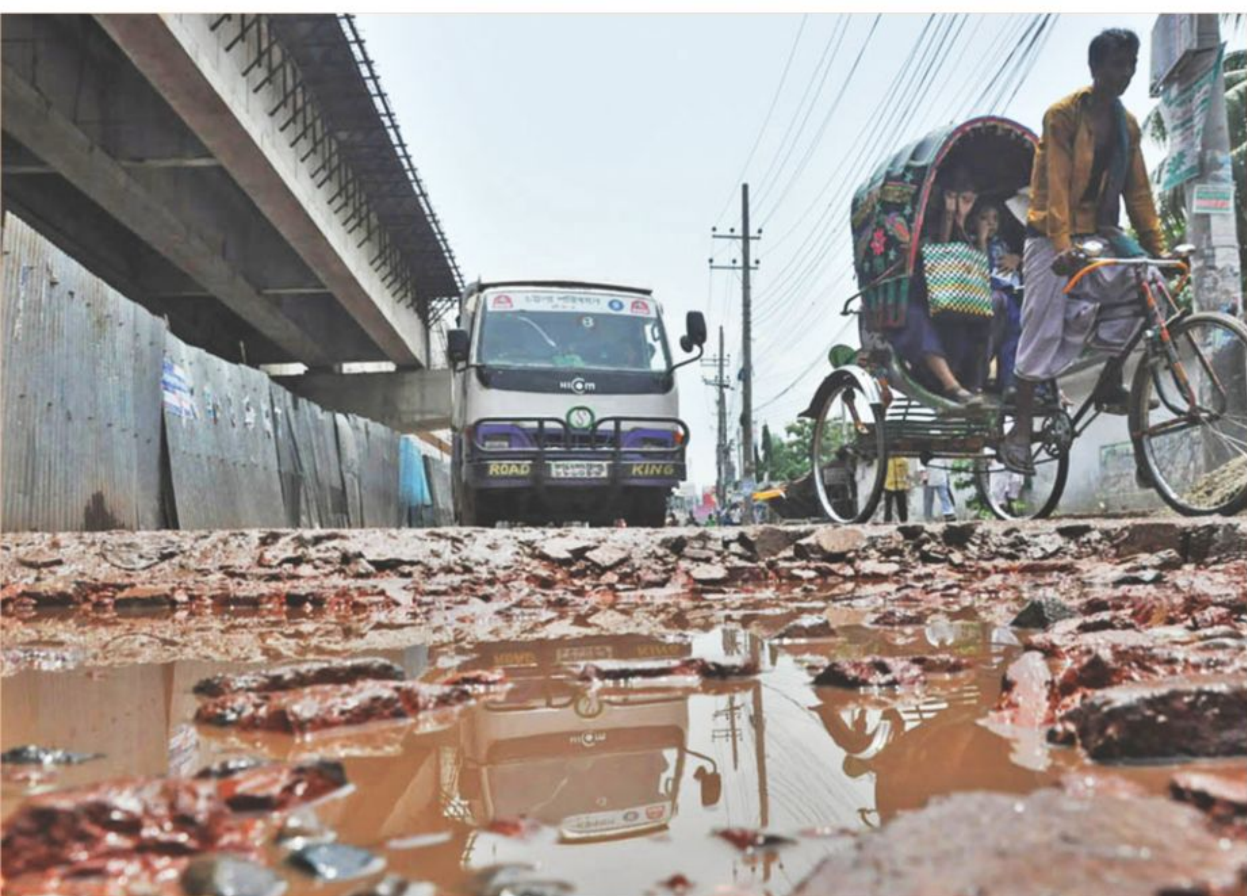
Streets of Chittagong city are in a dismal state. The photo was taken from Bahaddarhat yesterday.
