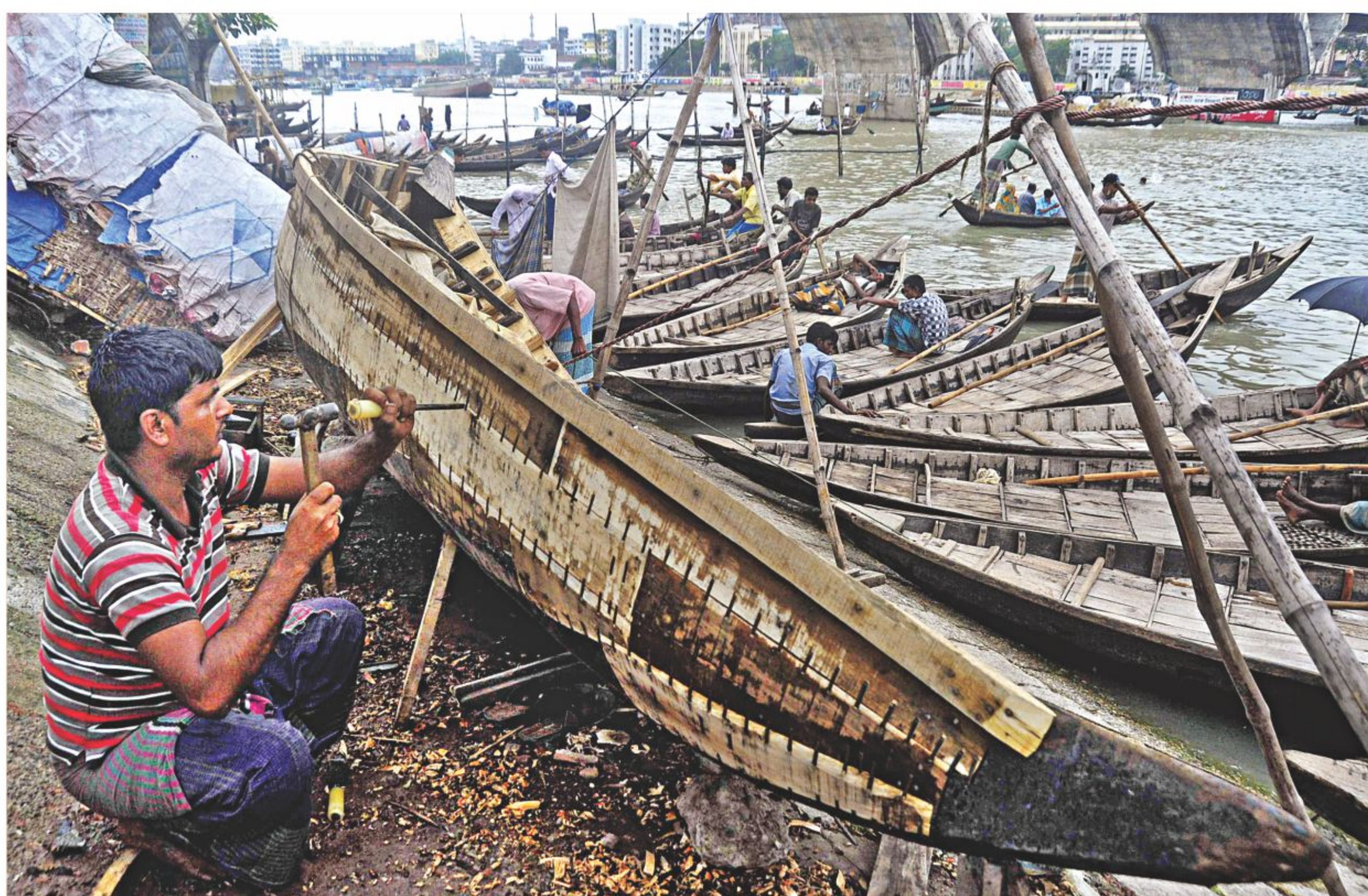
With the rainy season on, a boat owner repairs his vessel under the Buriganga Bridge-2 in the capital. The photo was taken yesterday.
