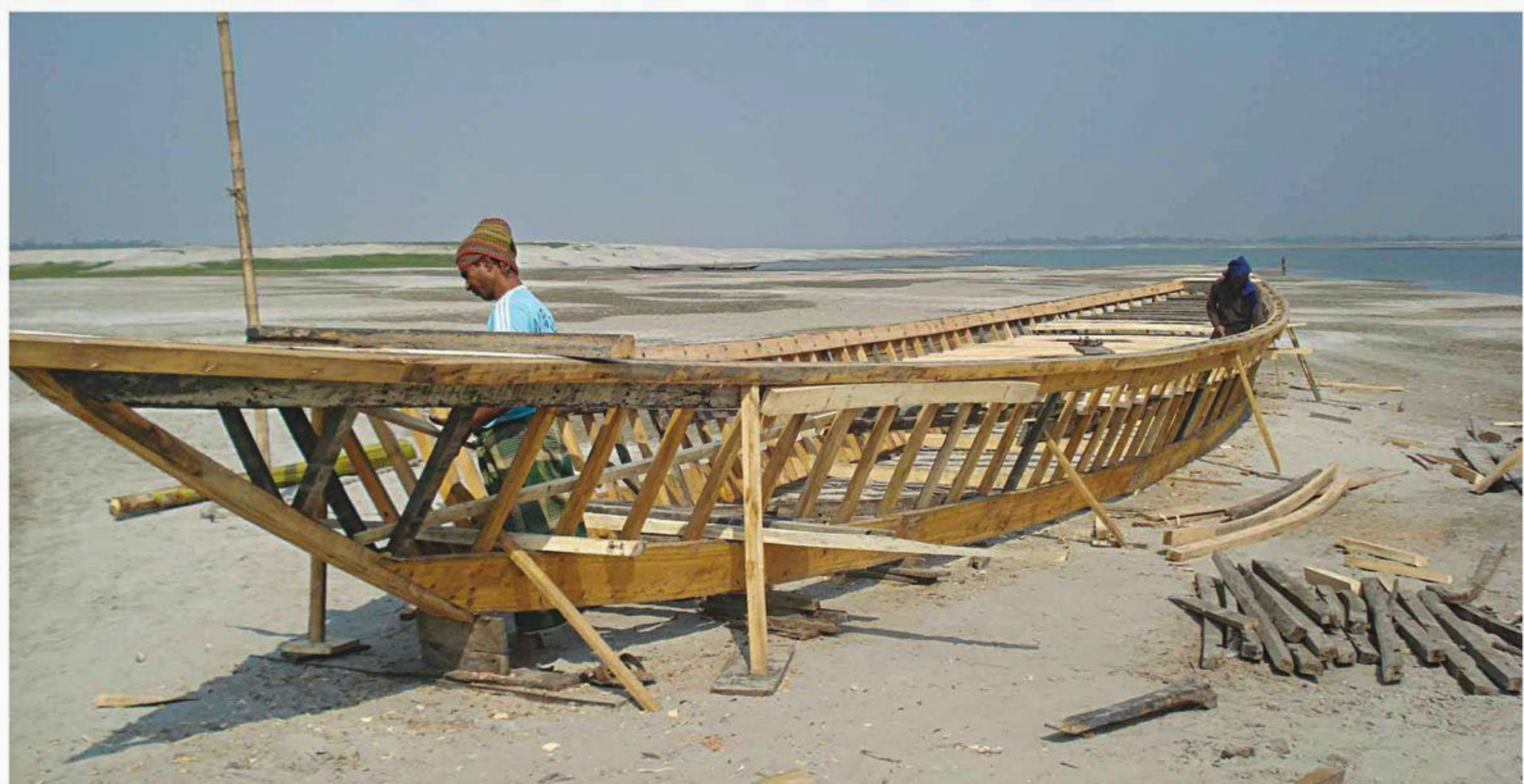
With the rains approaching, workers are busy making a wooden boat at Char Gabasa on the Jamuna basin in Bhupur upazila under Tangail district. Country boats serve as the main mode of transport in the area which gets flooded with the rise of water level in the mighty river. Most of the rural areas in the riverine country see similar situations during the rainy season.
