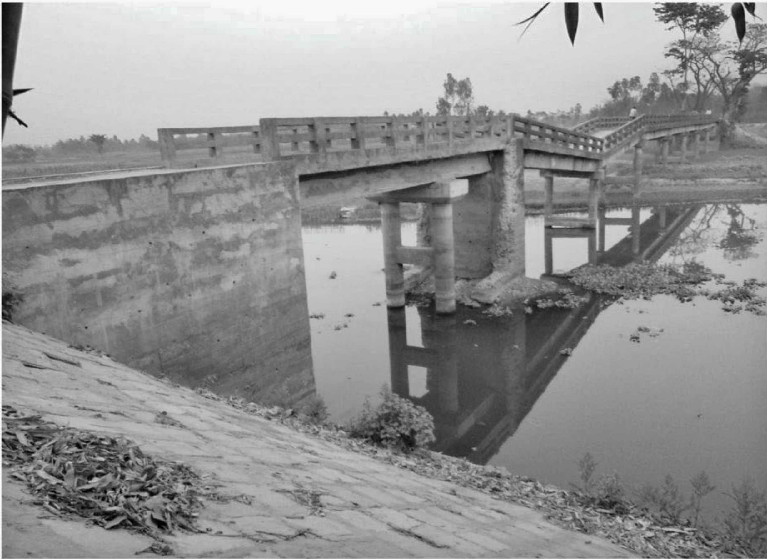
PHOTO: STAR PICTURE TELLS THE TALE: Naodanga Bridge over Baromashiya River in Phulbari upazila of Kurigram district has remained in a highly vulnerable position since subsidence of its two pillars over a year ago.
