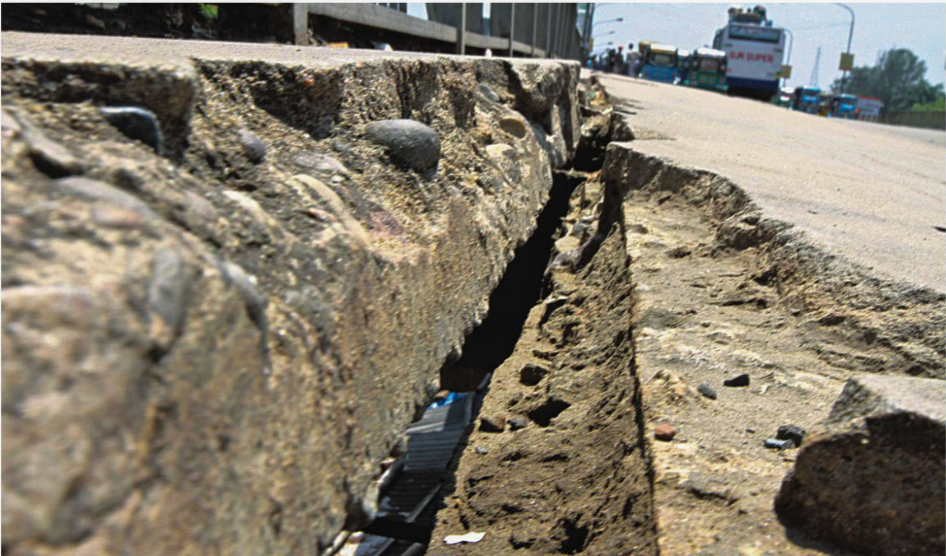
A gaping trench-like crack has appeared between the tarmac and the pavement of the first Buriganga Bridge in Postagola in the capital. The dangerous crack has been there for months but there have been no signs that the authorities concerned were trying to fix it.
