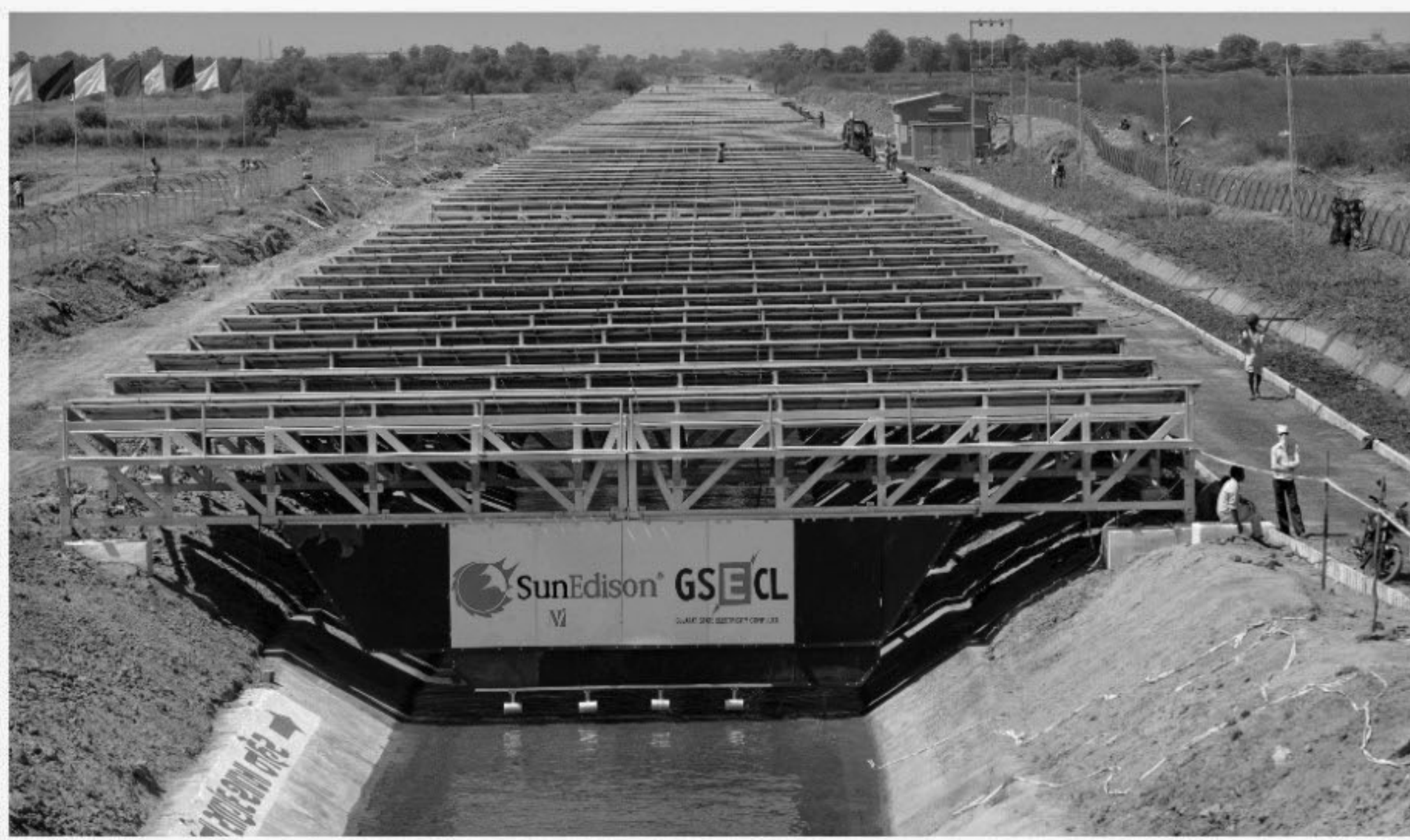
Indian workers give the finishing touches yesterday to India's first 1MW canal-top solar power plant at Chandrasana village of Mehsana district, some 45 kms from Ahmedabad on World Earth Day. This solar power plant on a 750 metre stretch of the Sanand Branch Canal of Sardar Sarovar Project will generate some 1.6 million units of clean electricity per year and will also prevent evaporation of some 90 lakh litres of water per year from the canal.
