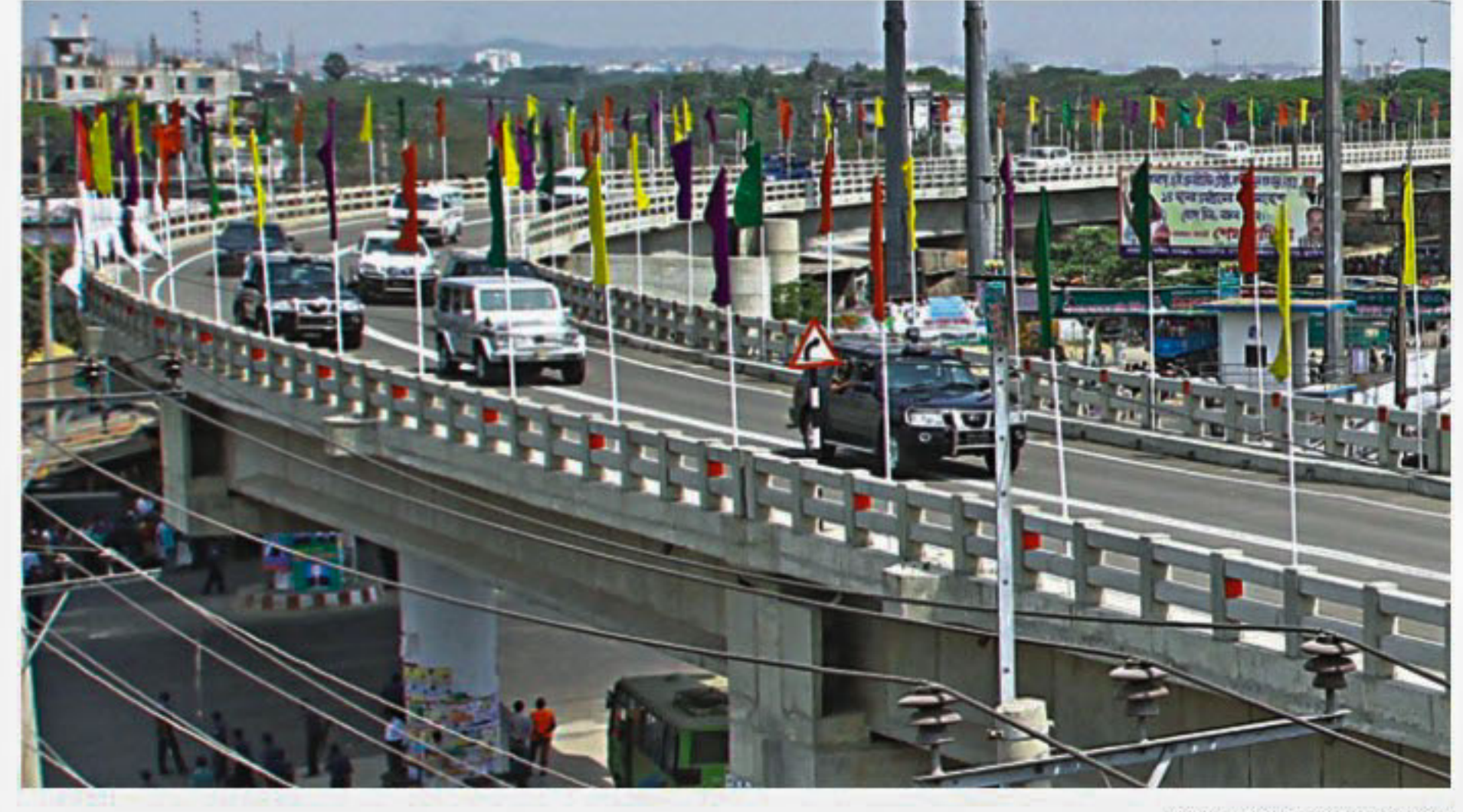
The first flyover in Chittagong promises to ease cargo transport in the port city.
