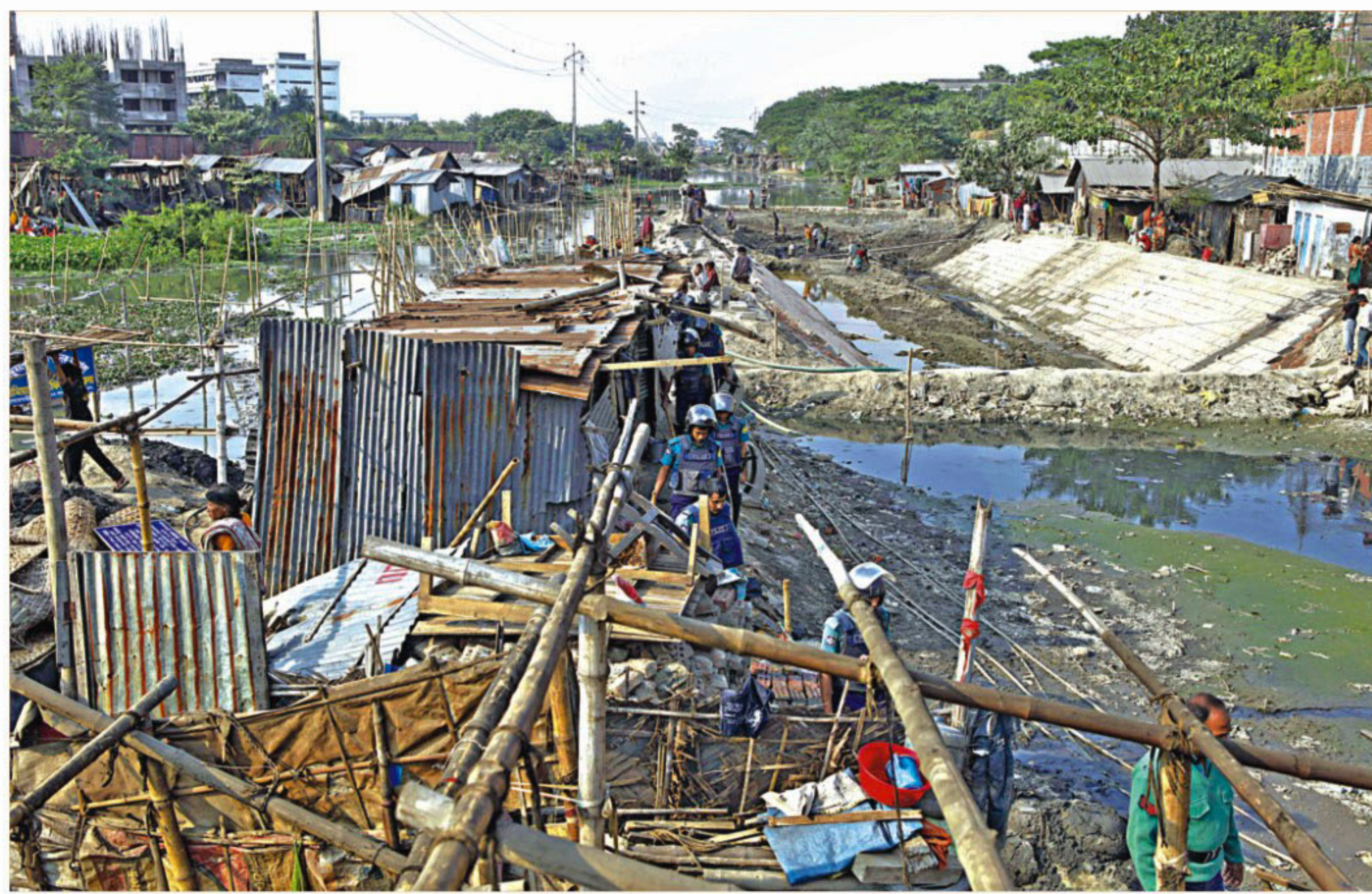
Remains of tin, wood and bamboo structures in Anandanagar slum in the city's Mirpur 14 yesterday after National Housing Authority carried out an eviction drive.
