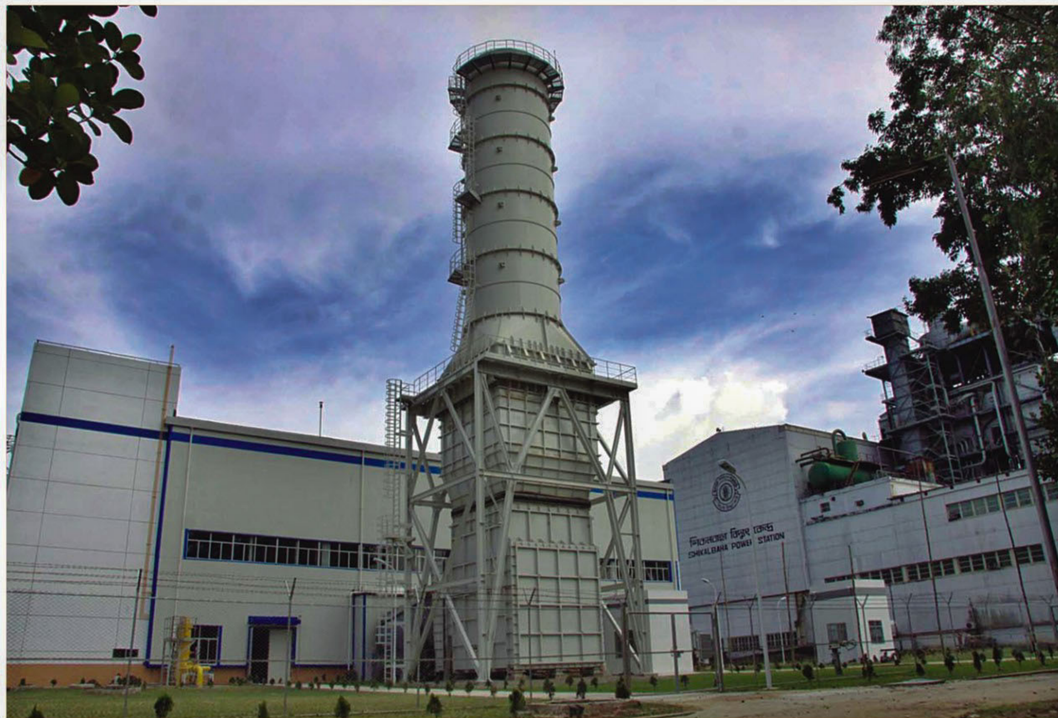
Shikalbaha Power Station.
