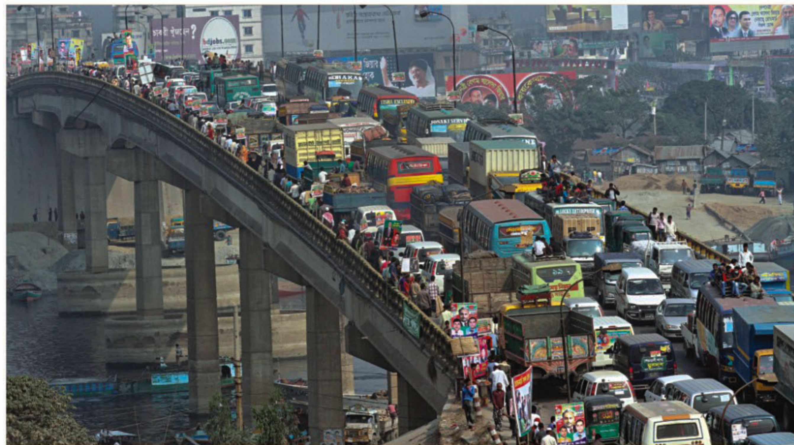
The opposition's road march towards Chittagong yesterday leaves a day-long gridlock at several places on Dhaka-Chittagong highway. The photo is of stationary vehicles on Kanchpur Bridge.
