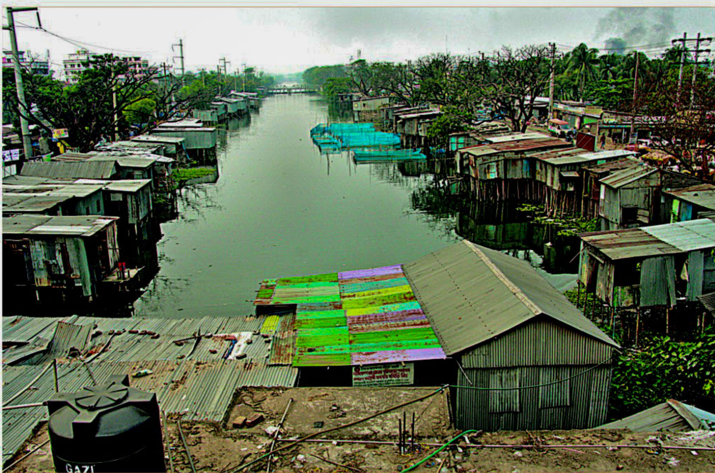
An influential quarter occupies the DND Canal in Narayanganj, builds structures on it and rents them out to people with the authorities concerned not caring much.
