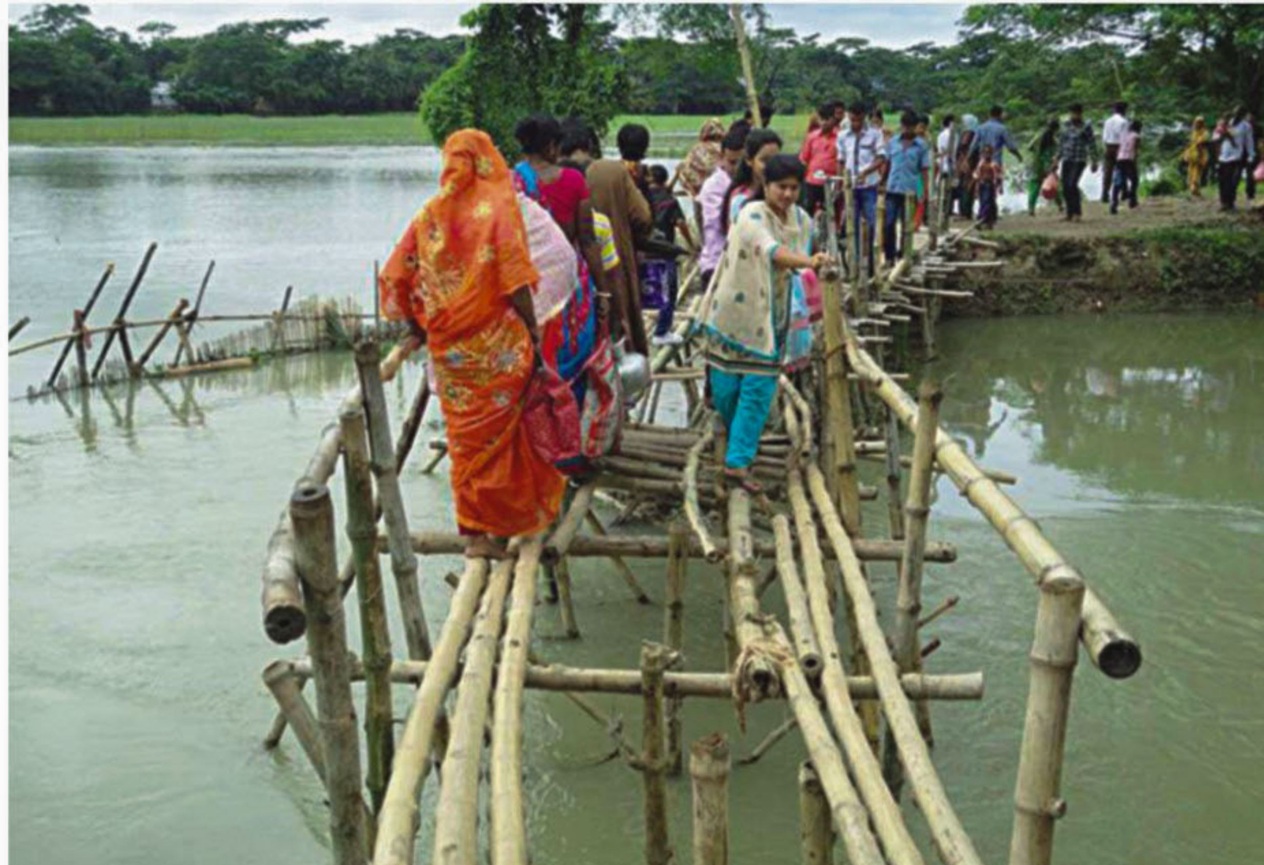
PHOTO: STAR People use a risky bamboo bridge to cross a water body at Jalkar on Charmuguria-Srinadi road in Shirkhara union under Madaripur Sadar upazila in absence of a concrete bridge there.
