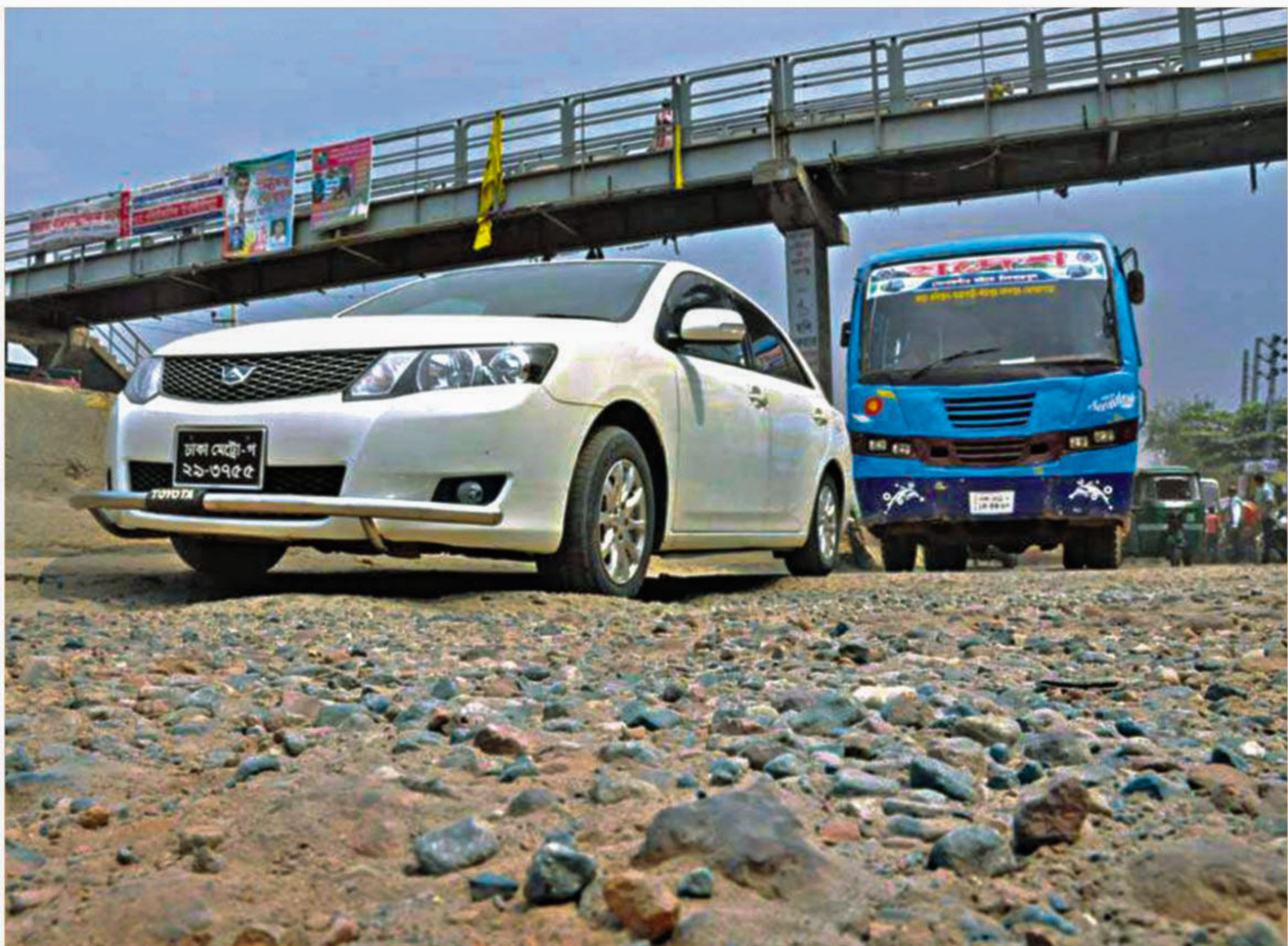
The Dhaka-Chittagong highway exposes rough stone chips inflicting serious inconvenience on travellers as its bitumen coating has eroded away. The photo was taken from Rayerbagh in the city yesterday.
