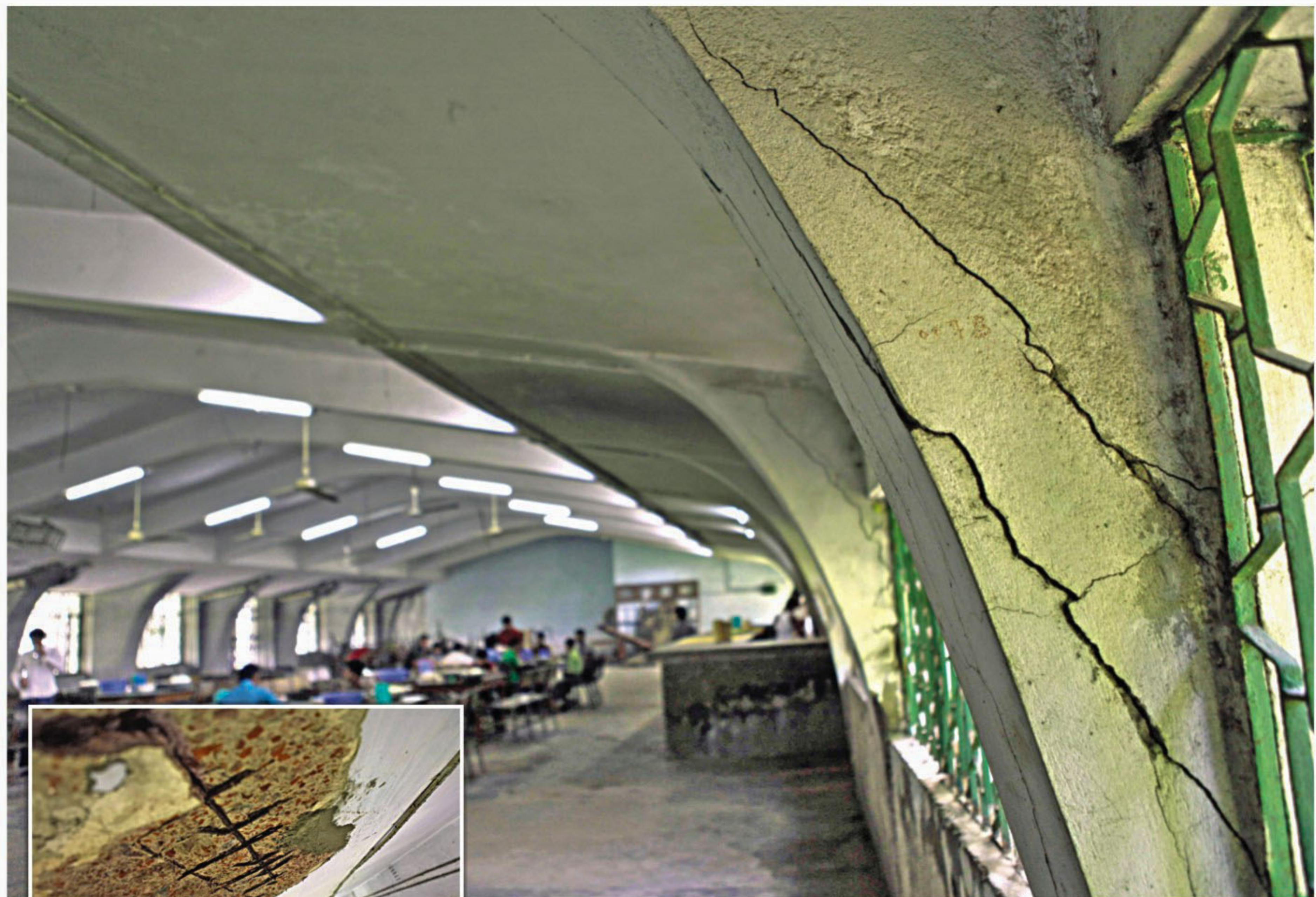
Cracked wall of Haji Muhammad Mushin Hall at Dhaka University. Inset, rods in the roof get exposed as chunks of plaster fell off earlier. The photos were taken yesterday. PHOTO: RASHED SHUMON
