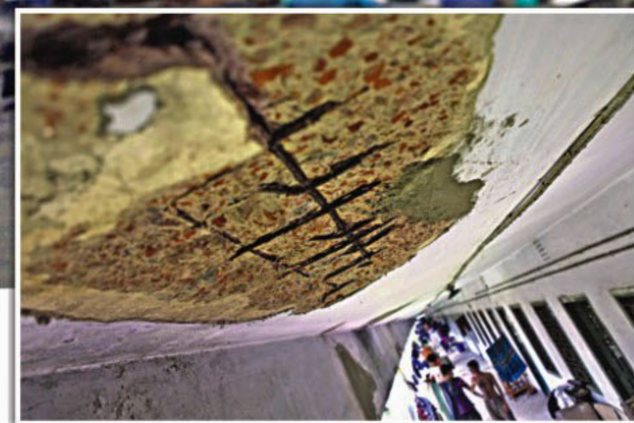
Cracked wall of Haji Muhammad Mushin Hall at Dhaka University. Inset, rods in the roof get exposed as chunks of plaster fell off earlier. The photos were taken yesterday. PHOTO: RASHED SHUMON
